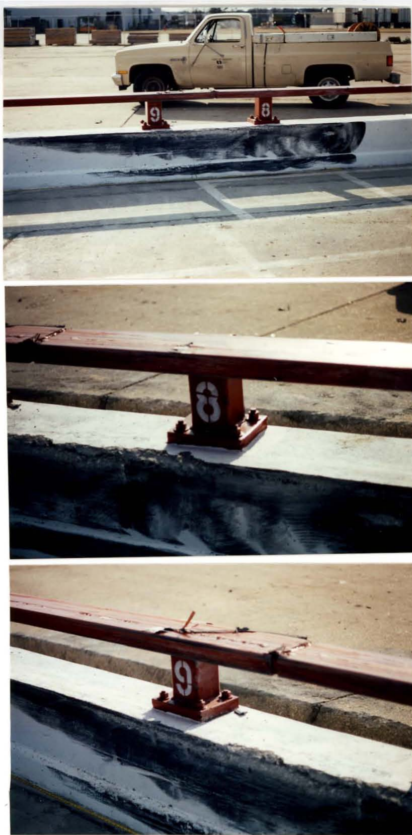
Figure 26. Bridge Rail Damage, Test MN-3.
