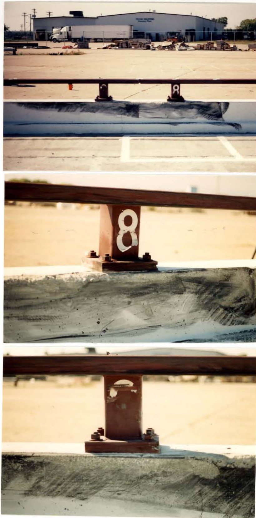
Figure 21. Bridge Rail Damage, Test MN-2.
