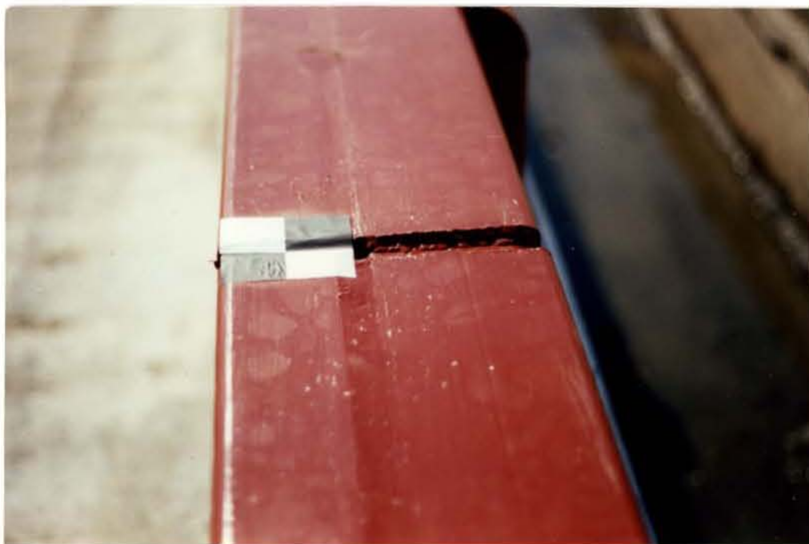
Figure 23. Retrofit of Minnesota Combination Bridge Rail for tests MN-3 and MN-4.
