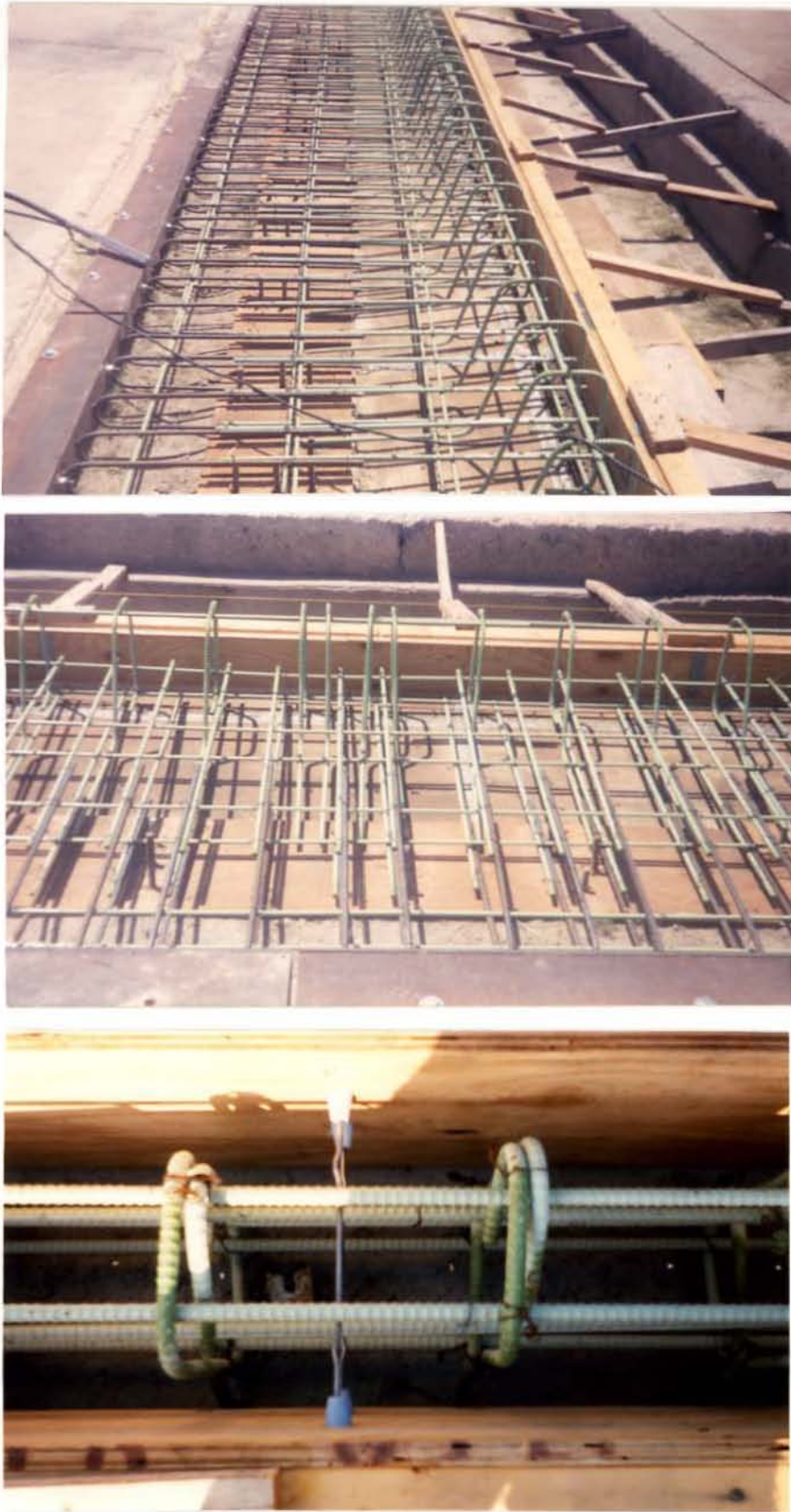
Figure 4. Reinforcement layout for bridge deck and parapet.
