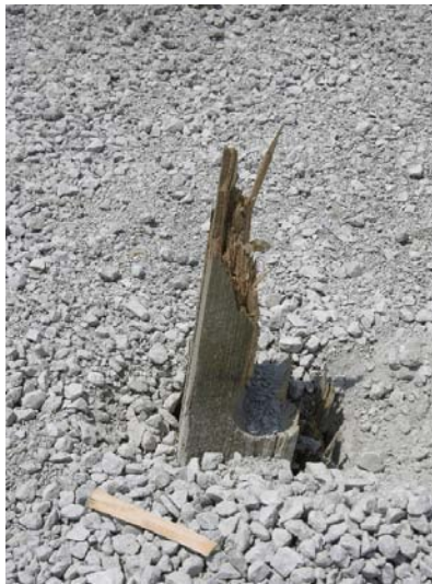
Figure 51. Post Nos. 6S through 8S Damage, Test SR-7
