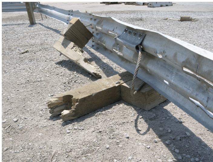
Figure 47. System Damage, Test SR-7
