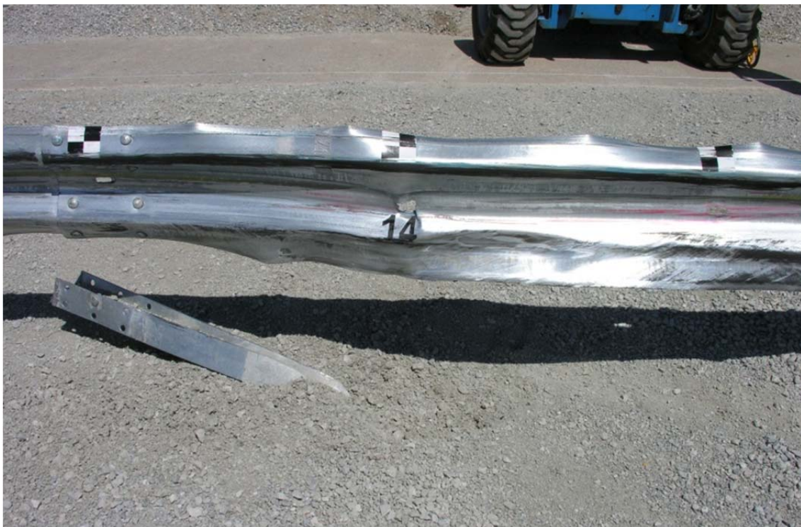
Figure 40. Guardrail Damage between Post Nos. 13 and 17, Test No. MGSNB-1
