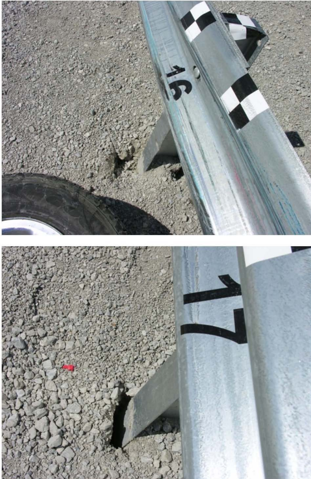
Figure 43. Post Damage between Post Nos. 16 and 17, Test No. MGSNB-1
