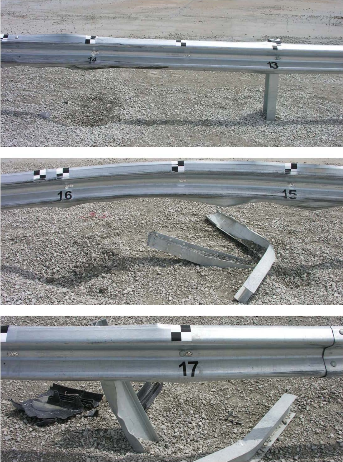
Figure 55. Guardrail Damage between Posts 13 and 17, Test No. MGSNB-2
