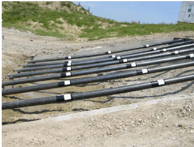
Figure 29. Culvert Grate System Damage, Test KSCG-1
