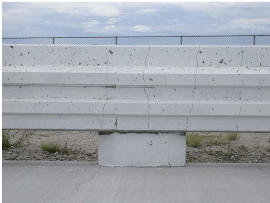
Figure 19. NDOR's TL-5 Aesthetic Open Concrete Bridge Rail
