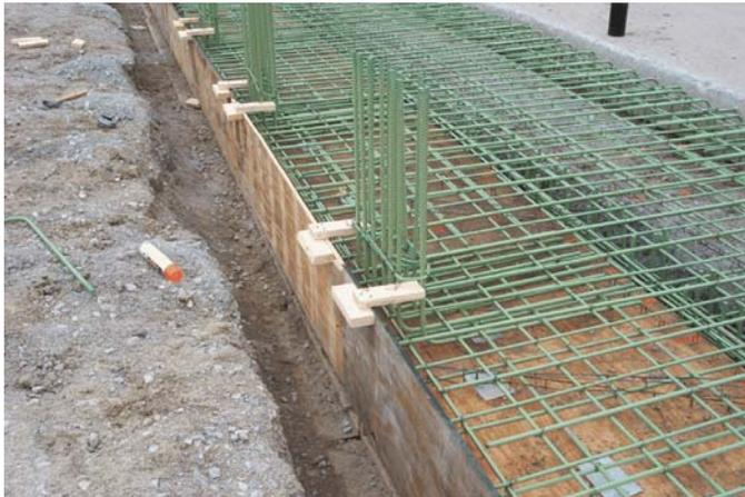
Figure 14. Bridge Deck Rebar Reinforcement
