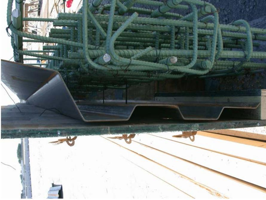
Figure 16. NDOR's TL-5 Aesthetic Open Concrete Bridge Rail Rebar Reinforcement
