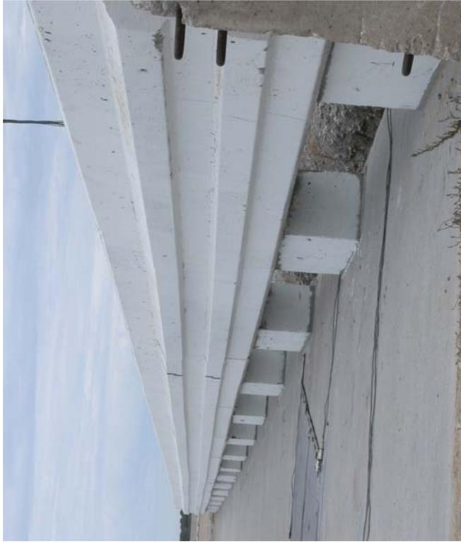
Figure 18. NDOR's TL-5 Aesthetic Open Concrete Bridge Rail
