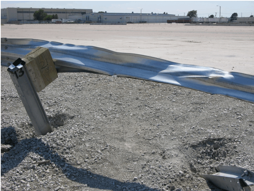
Figure 28. System Damage, Test No. MGSAS-1
