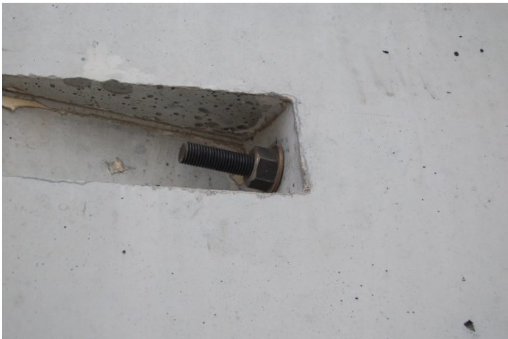
Figure 15. Barrier Connection Joints, Test No. KSFRP-1
