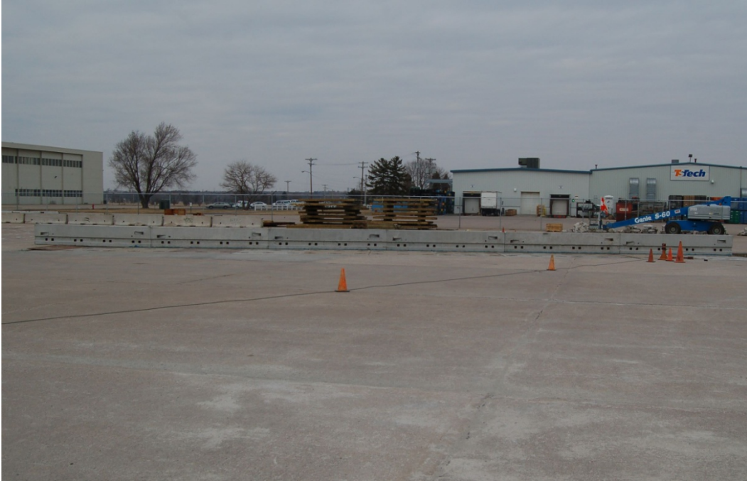
Figure 12. Test Installation, Test No. KSFRP-1
