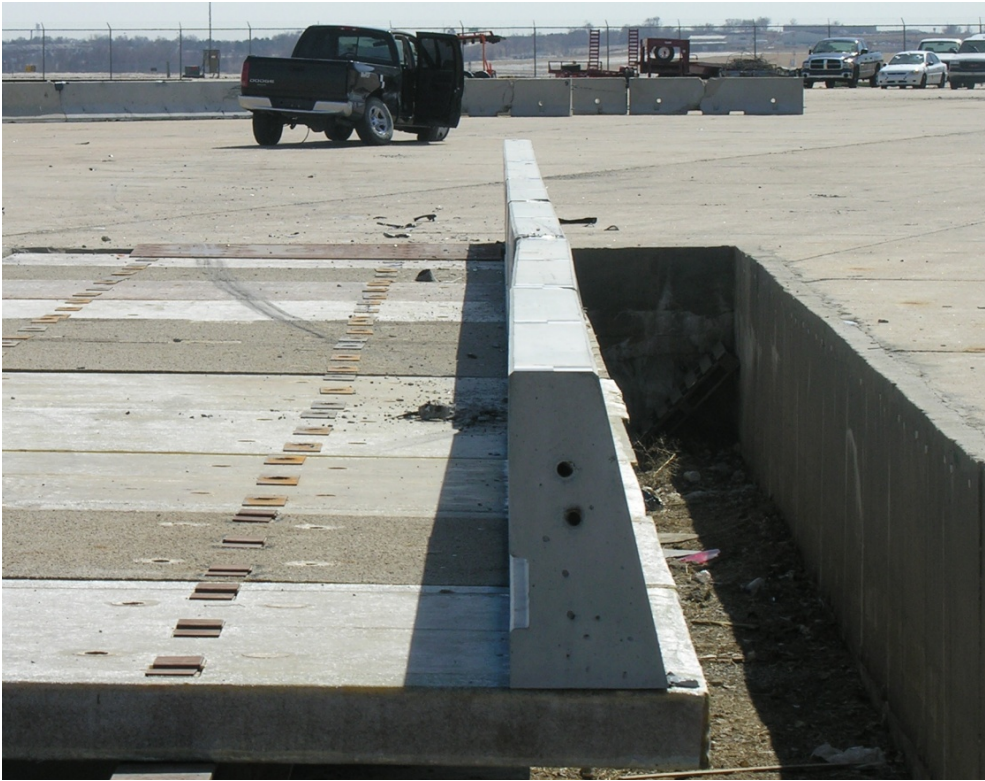
Figure 28. System Damage, Test No. KSFRP-1
