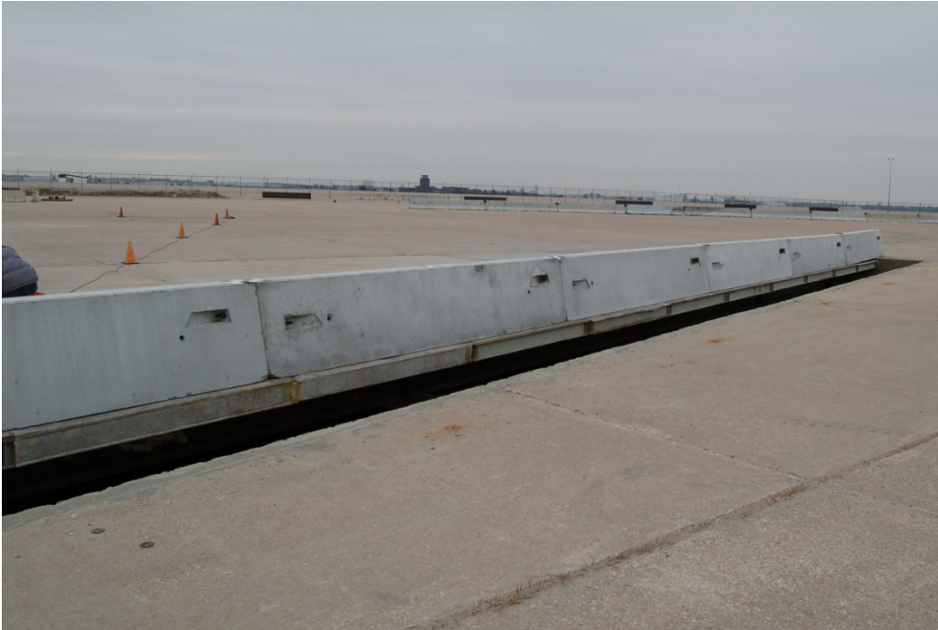
Figure 13. Test Installation, Test No. KSFRP-1
