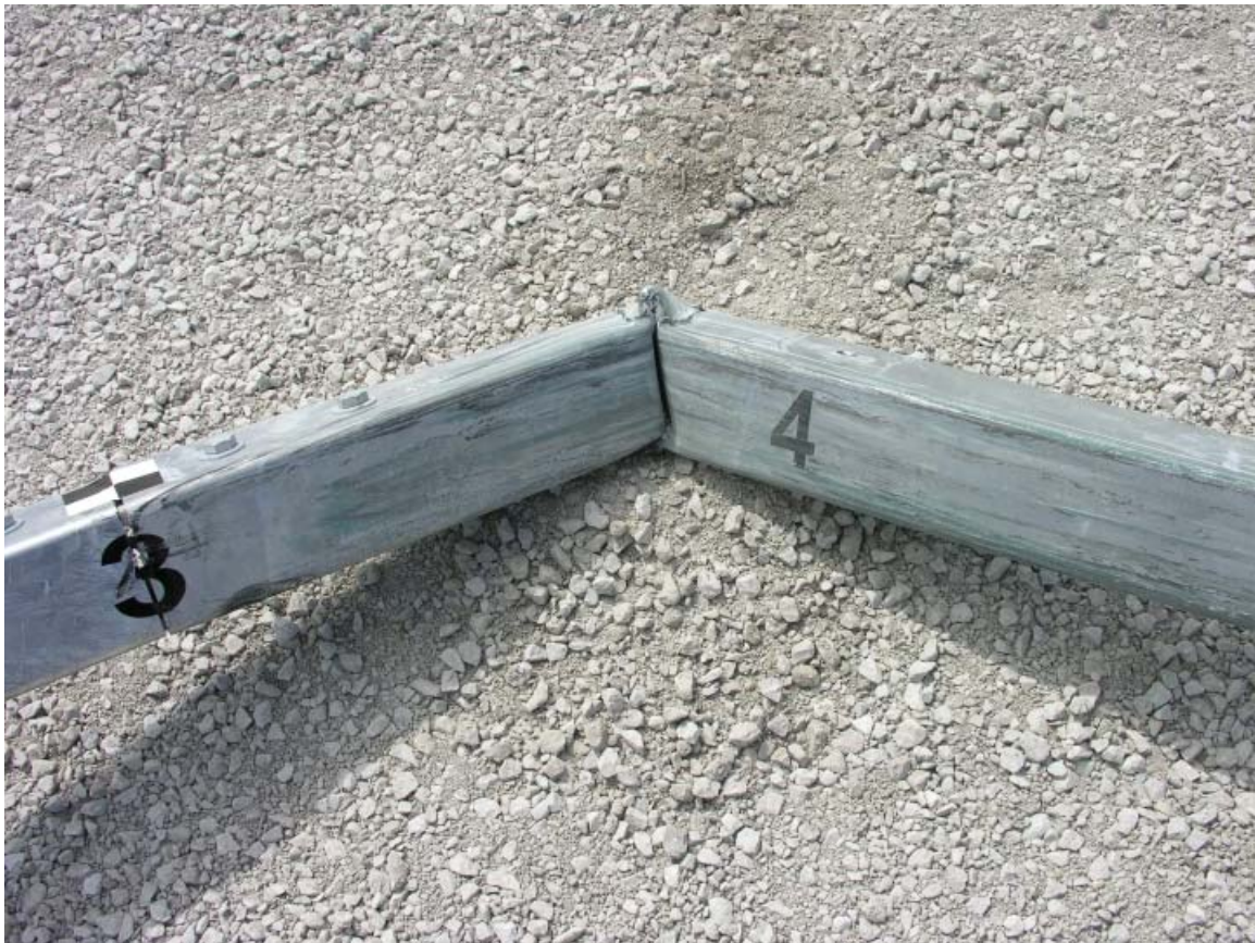
Figure 254. Barrier Damage, Test No. NYBBT-8
