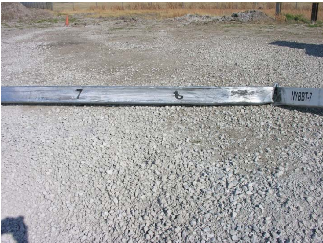
Figure 212. Barrier Damage, Test No. NYBBT-7
