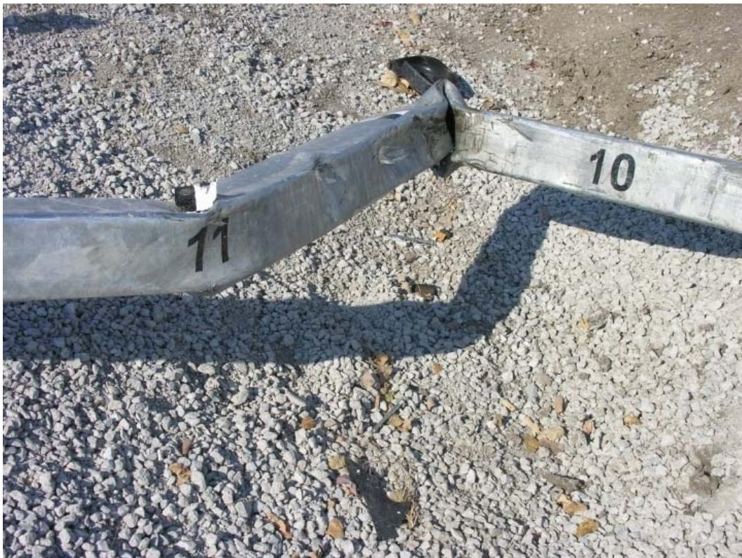
Figure 213. Barrier Damage, Test No. NYBBT-7
