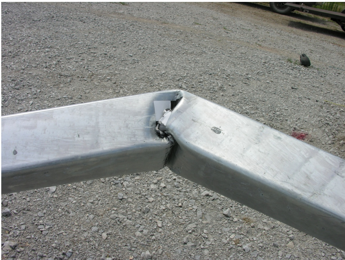
Figure 282. Barrier Damage, Test No. NYBBT-9
