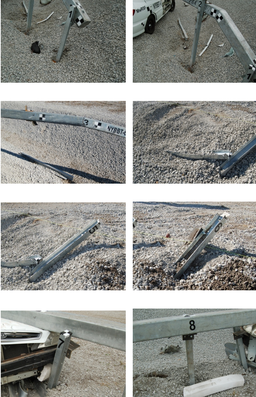
Figure 198. Post Nos. 1 through 8 Damage, Test No. NYBBT-6
