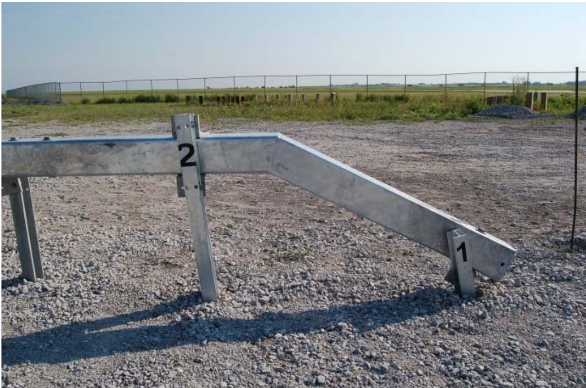
Figure 156. Barrier Damage, Test No. NYBBT-5
