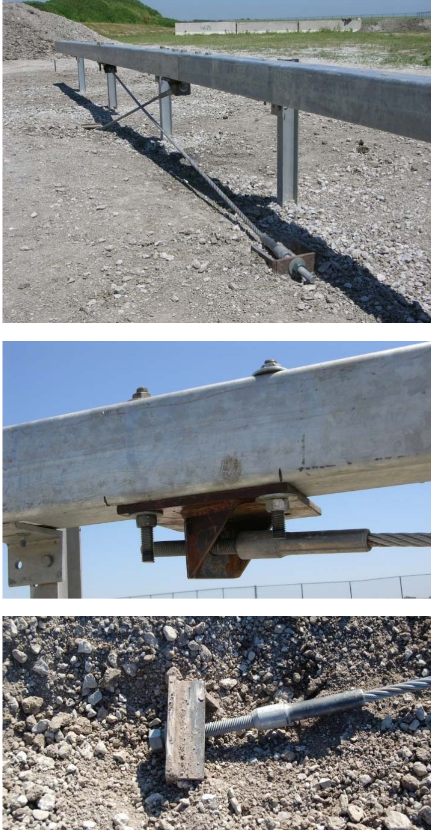
Figure 113. NYBBT-4 System Details
