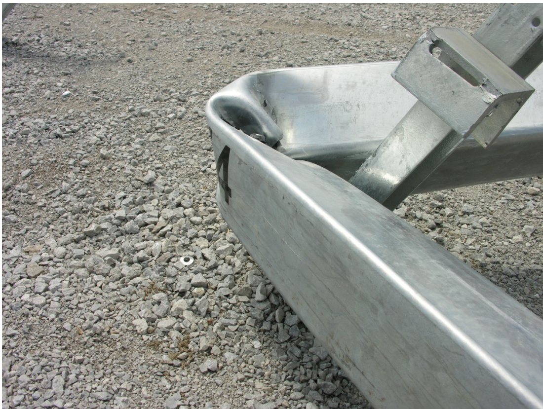
Figure 283. Barrier Damage, Test No. NYBBT-9
