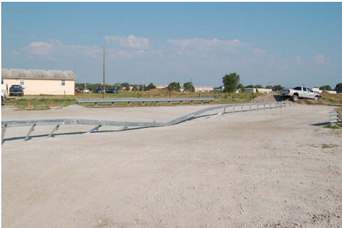
Figure 155. Barrier Damage, Test No. NYBBT-5
