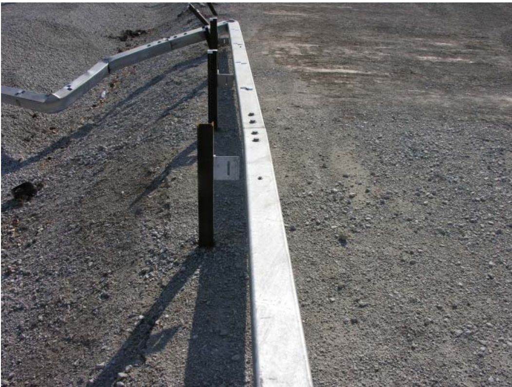
Figure 211. Barrier Damage, Test No. NYBBT-7
