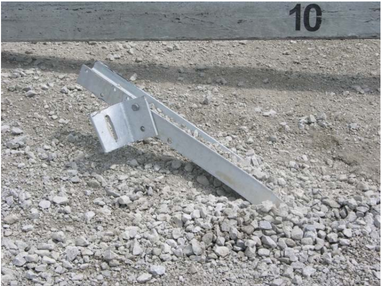
Figure 161. Post Nos. 9 and 10 Damage, Test No. NYBBT-5
