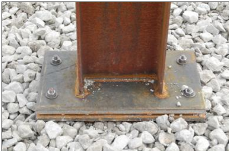
Figure 26. Assembled Fracturing Bolt (Slipbase) Design
