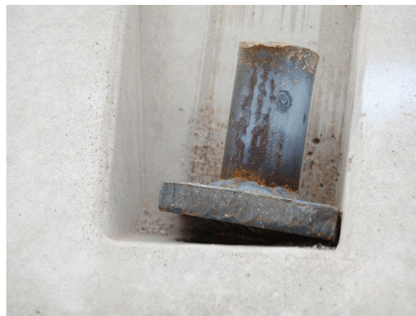
Barrier No. 2 Traffic Side Upstream
