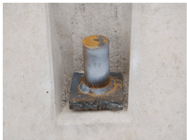
Barrier No. 4 Traffic Side Downstream
