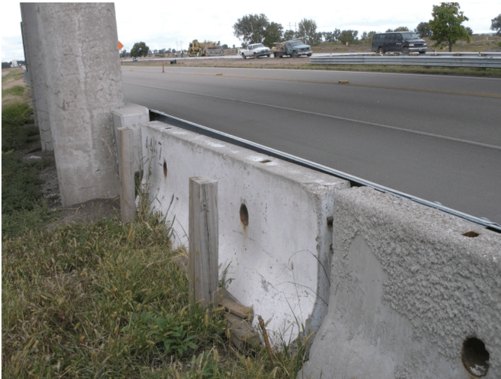
Figure B-8. Nebraska Temporary Barrier Transitions
