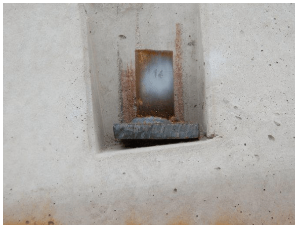
Barrier No. 3 Traffic Side Upstream
