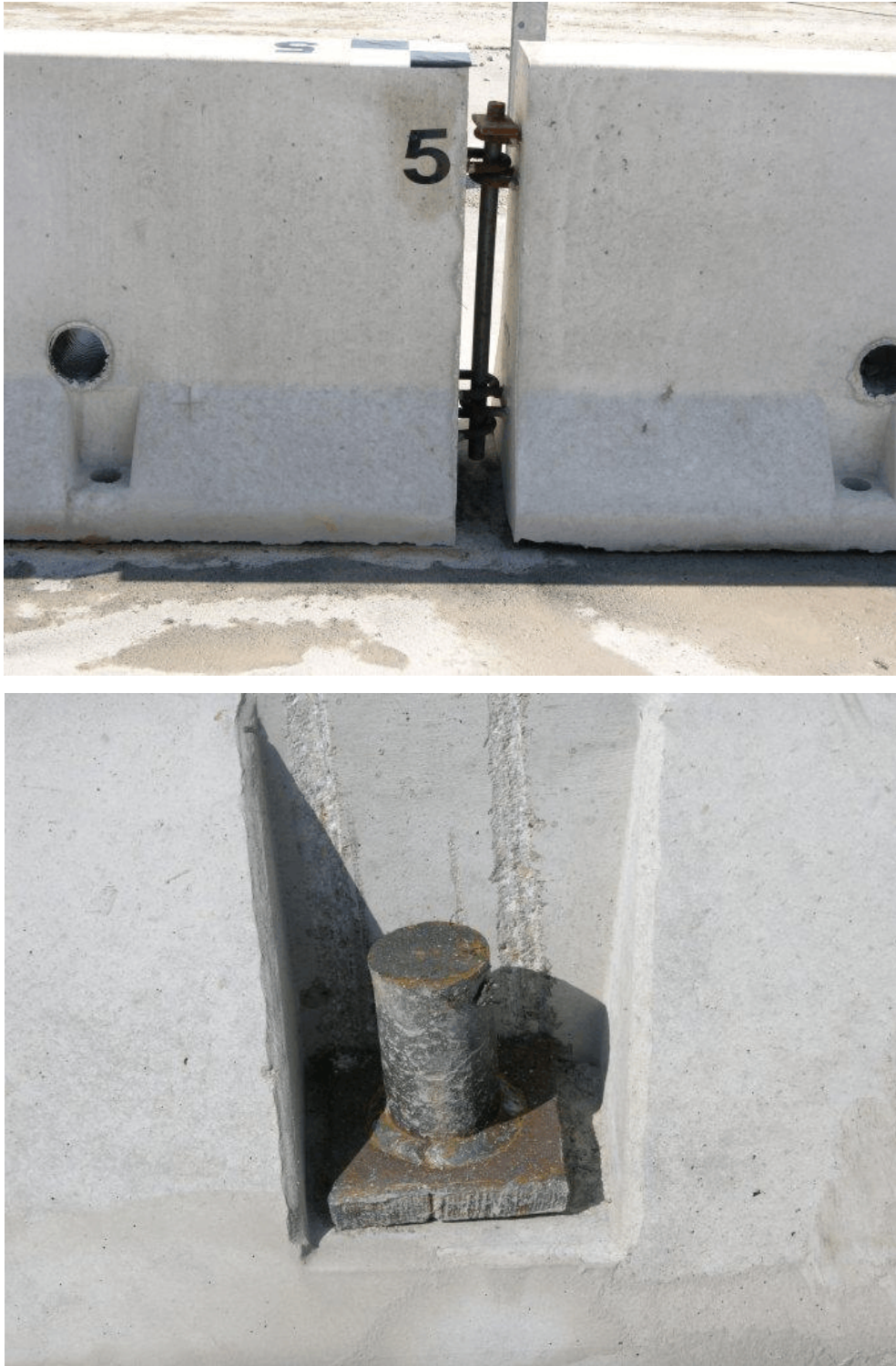
Figure 23. Temporary Concrete Barrier to Permanent Concrete Barrier Transition, Test No. TCBT-1 and TCBT-2
