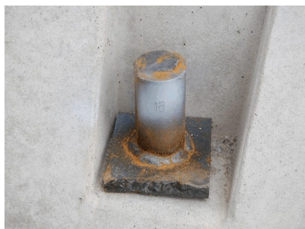
Barrier No. 4 Non-Traffic Side Downstream
