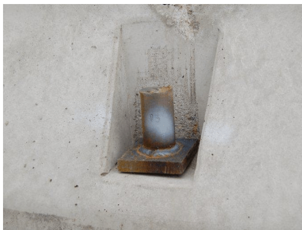
Barrier No. 3 Non-Traffic Side Downstream
