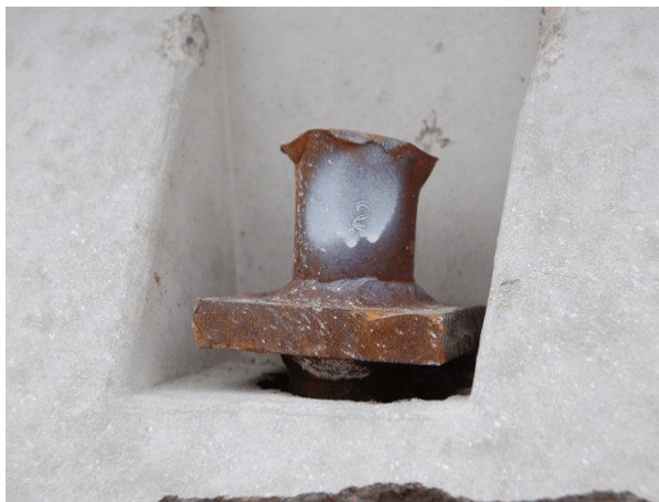
Barrier No. 1 Traffic Side Midspan
