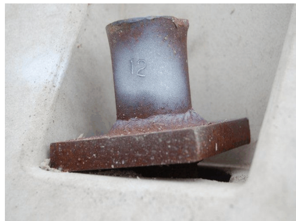
Barrier No. 2 Non-Traffic Side Upstream
