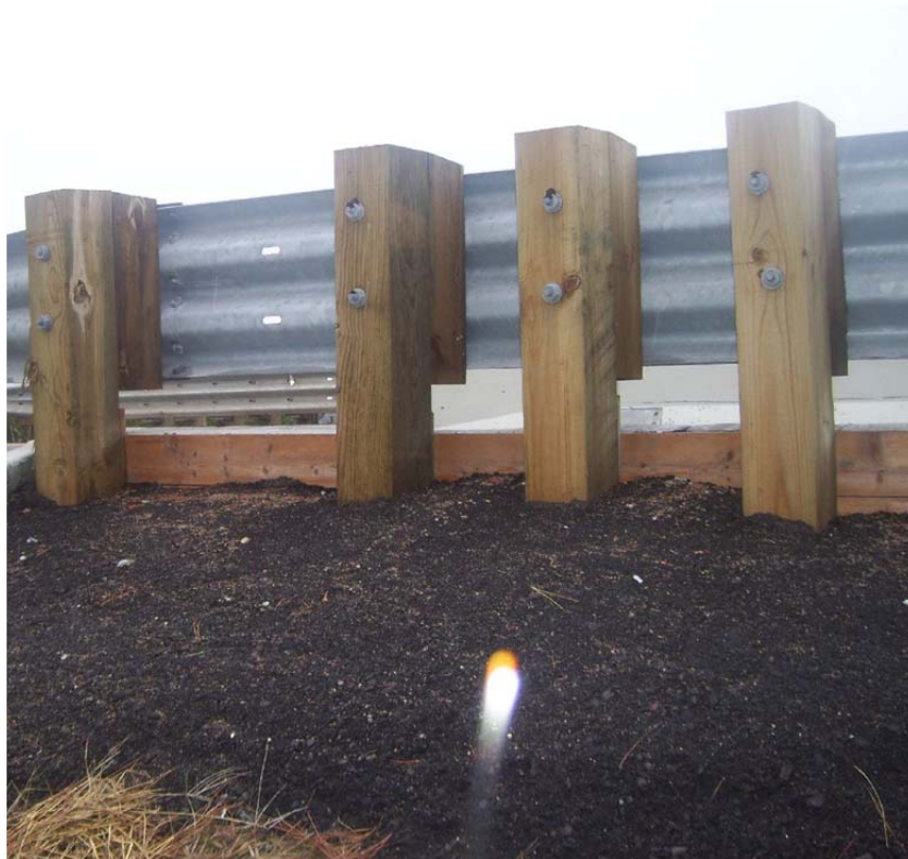
Figure 85. Asphalt Placement on Sloped Terrain
