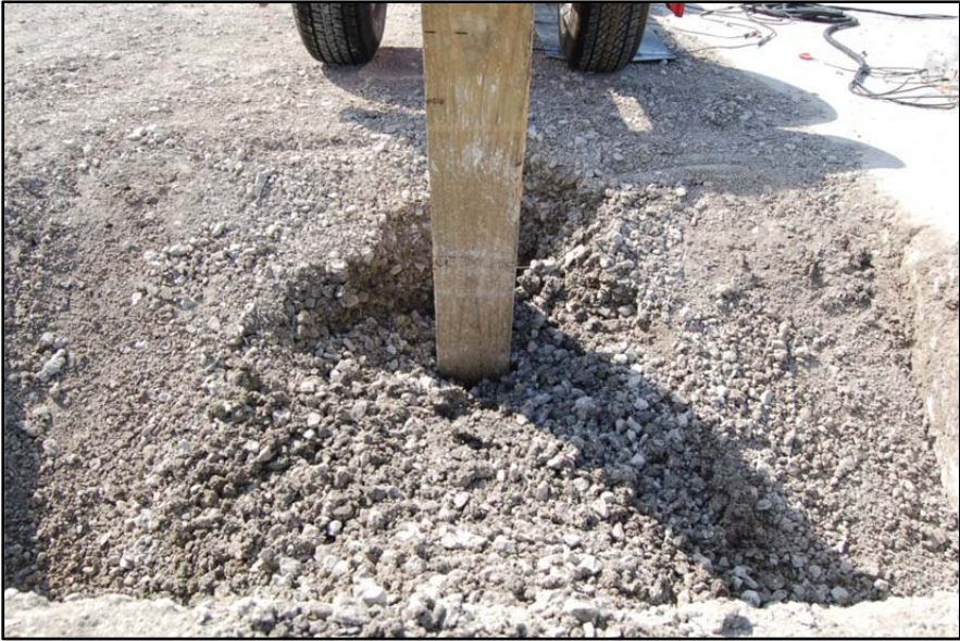
Post After Impact – Soil Displacement
