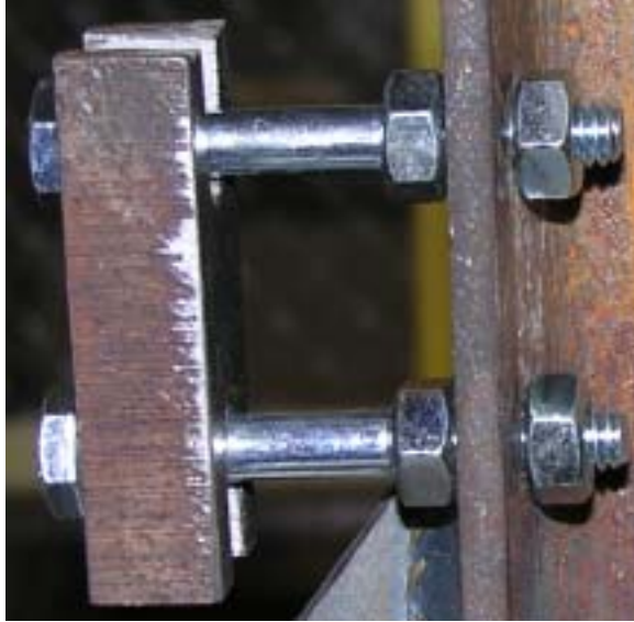
Figure 25. U-Bolt Clip, Style 2
