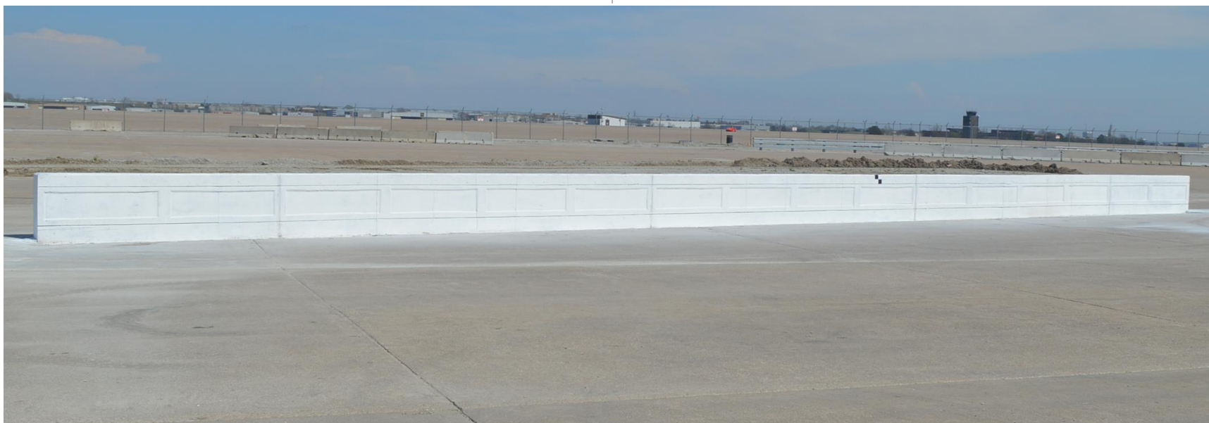
Figure 35. System Damage, Test No. H34BR-1
