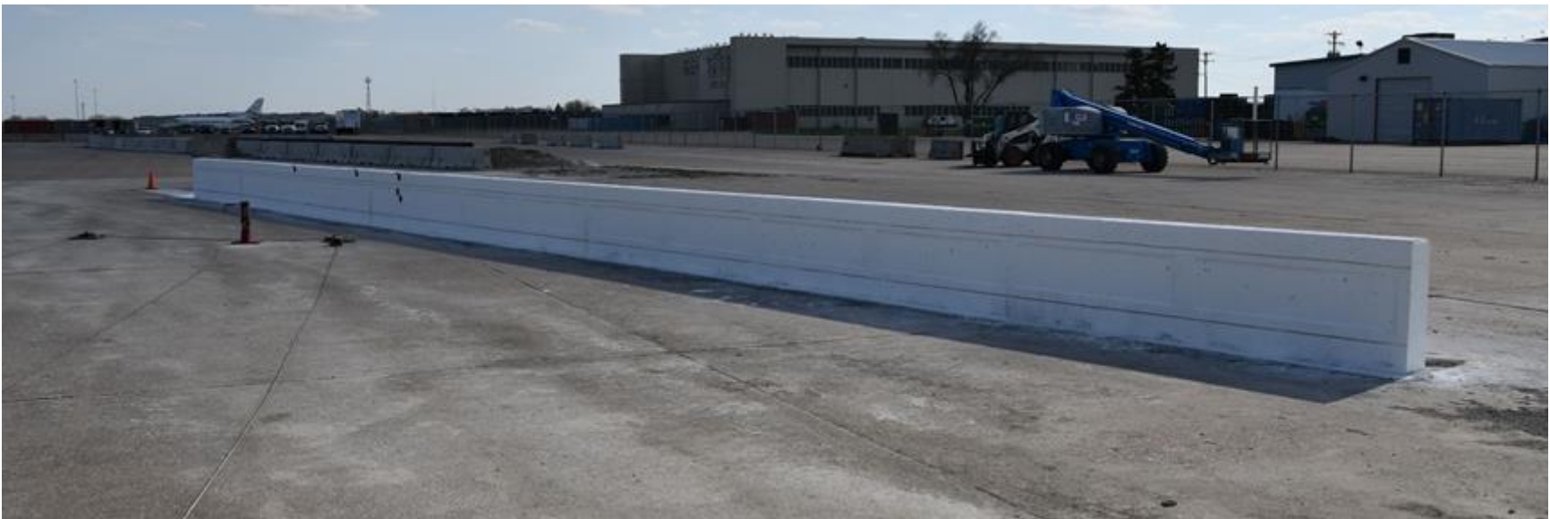
Figure 15. Test Installation Photographs, Test Nos. H34BR-1 and H34BR-2
