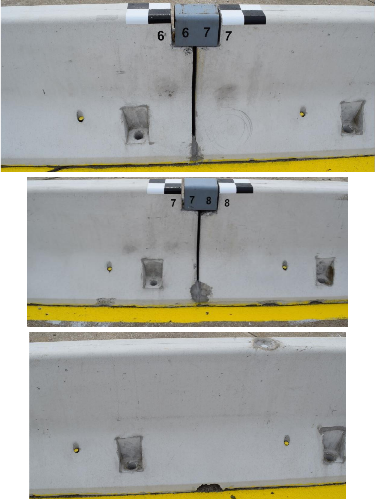
Figure 17. PCB Traffic-Side Pin Anchor Recesses, Test No. NJPCB-7
