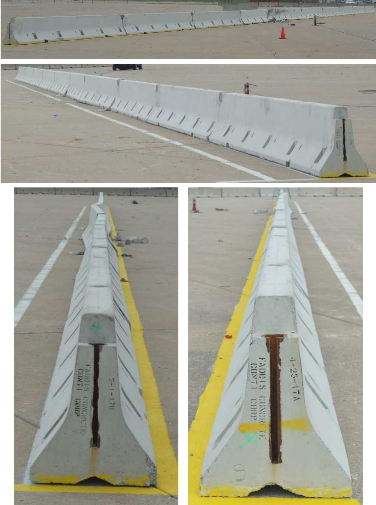
Figure 33. System Damage – Front, Back, Upstream and Downstream Views, Test No. NJPCB-7
