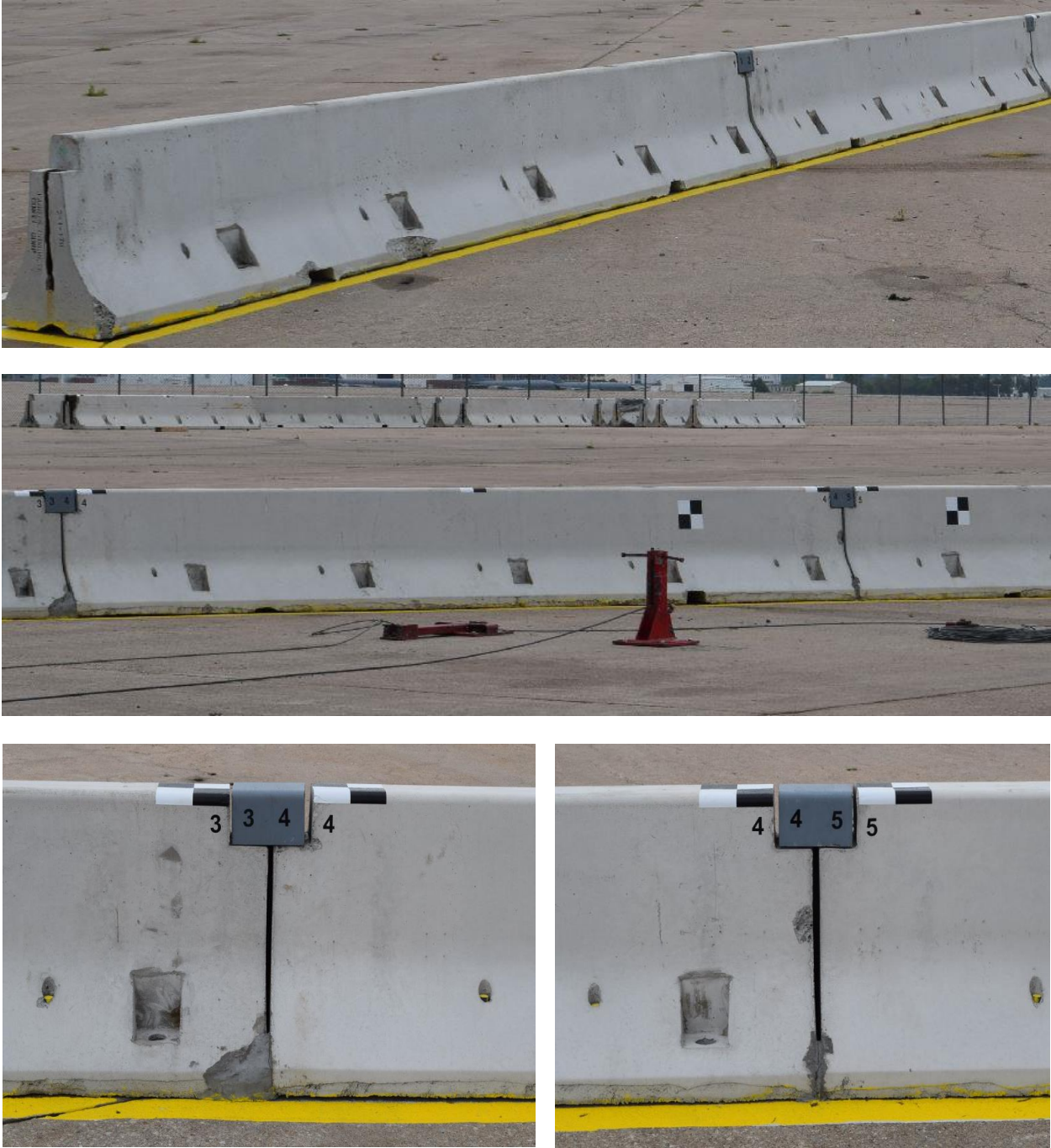
Figure 18. Grout at Toes between PCBs, Test No. NJPCB-7
