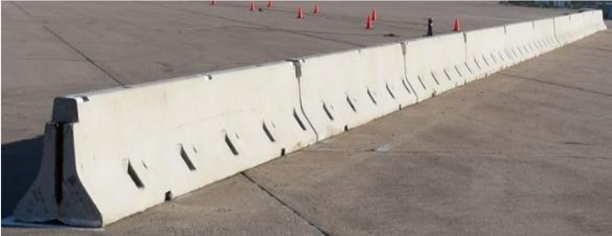
Figure 15. NJDOT PCB with Free-Standing Configuration Test Installation, Test No. NJPCB-3
