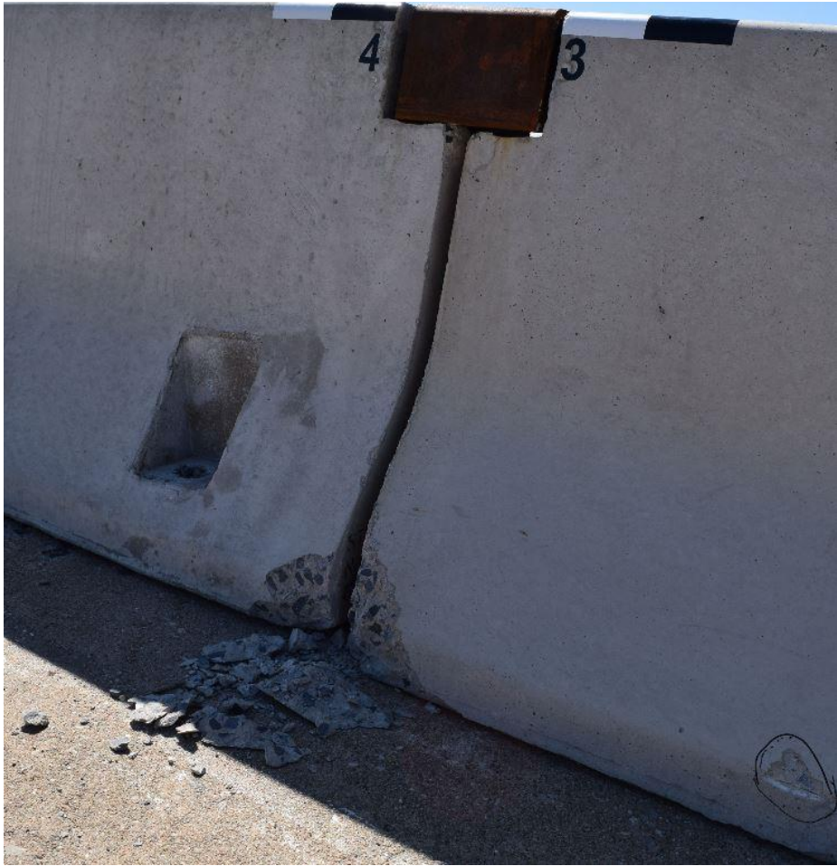
Figure 30. Barrier No. 3 Traffic-side and Back-side Damage, Test No. NJPCB-3
