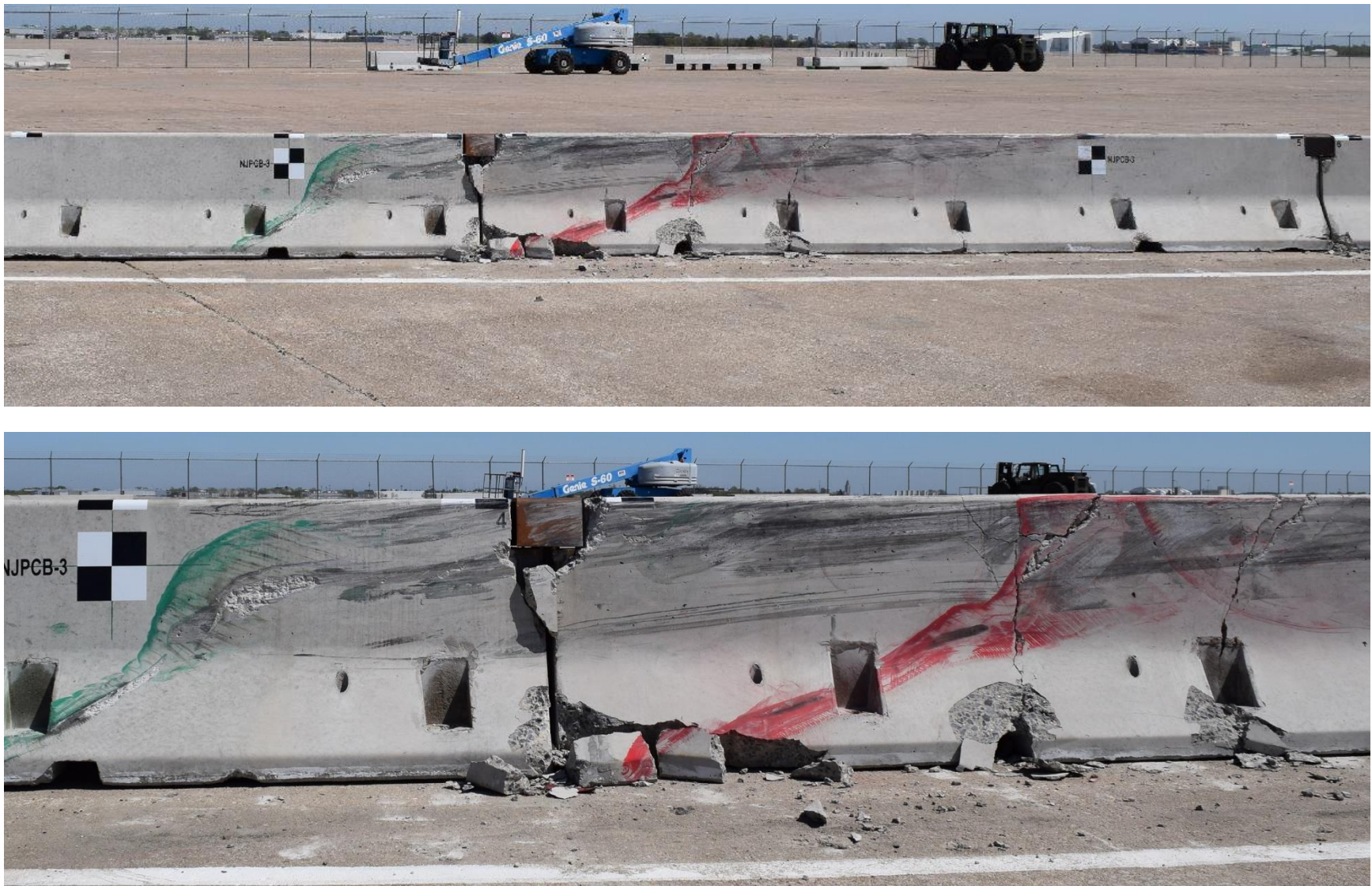
Figure 31. Barrier Nos. 4 and 5 Damage, Test No. NJPCB-3
