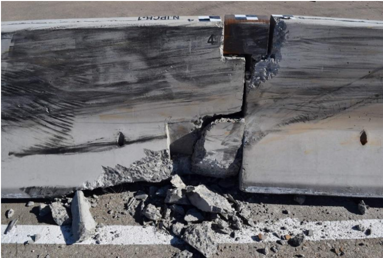
Figure 31. System Damage at Impact Location, Test No. NJPCB-1
