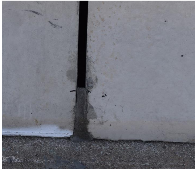
Figure 18. Grout at Toes between PCBs, Test No. NJPCB-1
