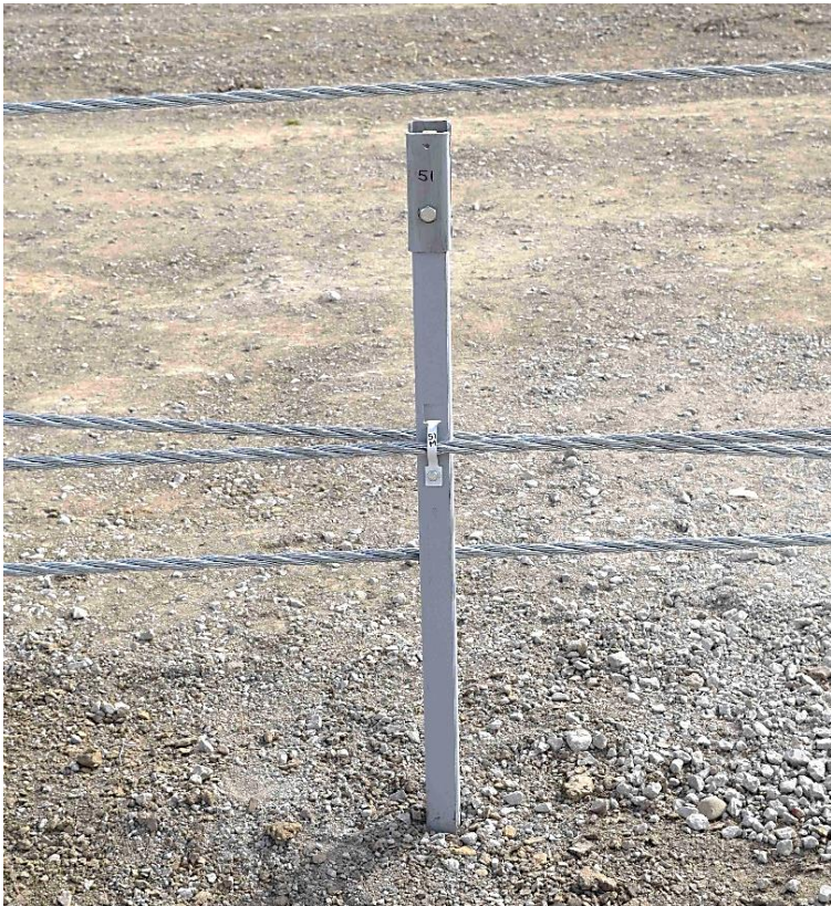
Figure 83. Post No. 51 Damage, Test No. MWP-9 99
