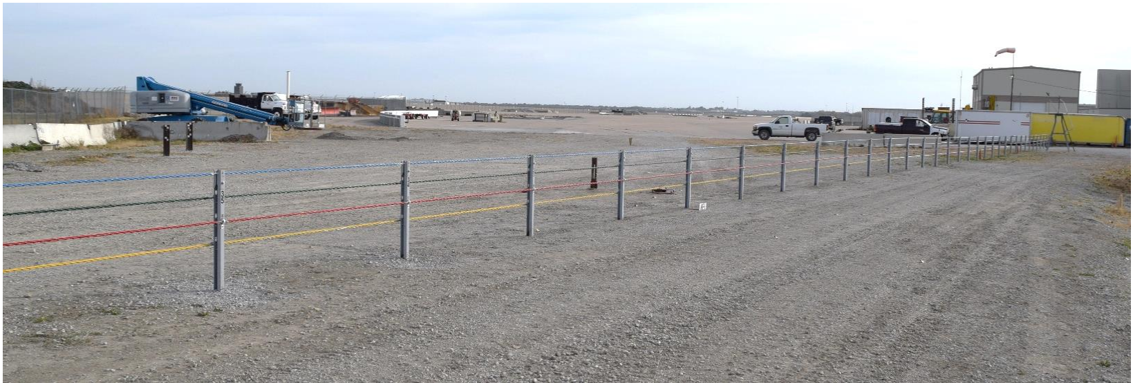
Figure 27. System Installation, Test No. MWP-9
