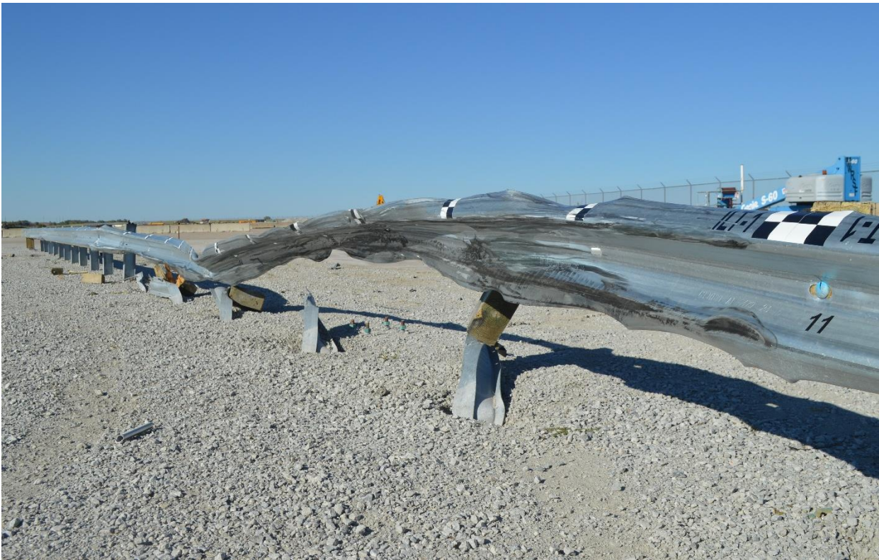
Figure 113. Midwest Guardrail System Damage, Test No. ILT-1
