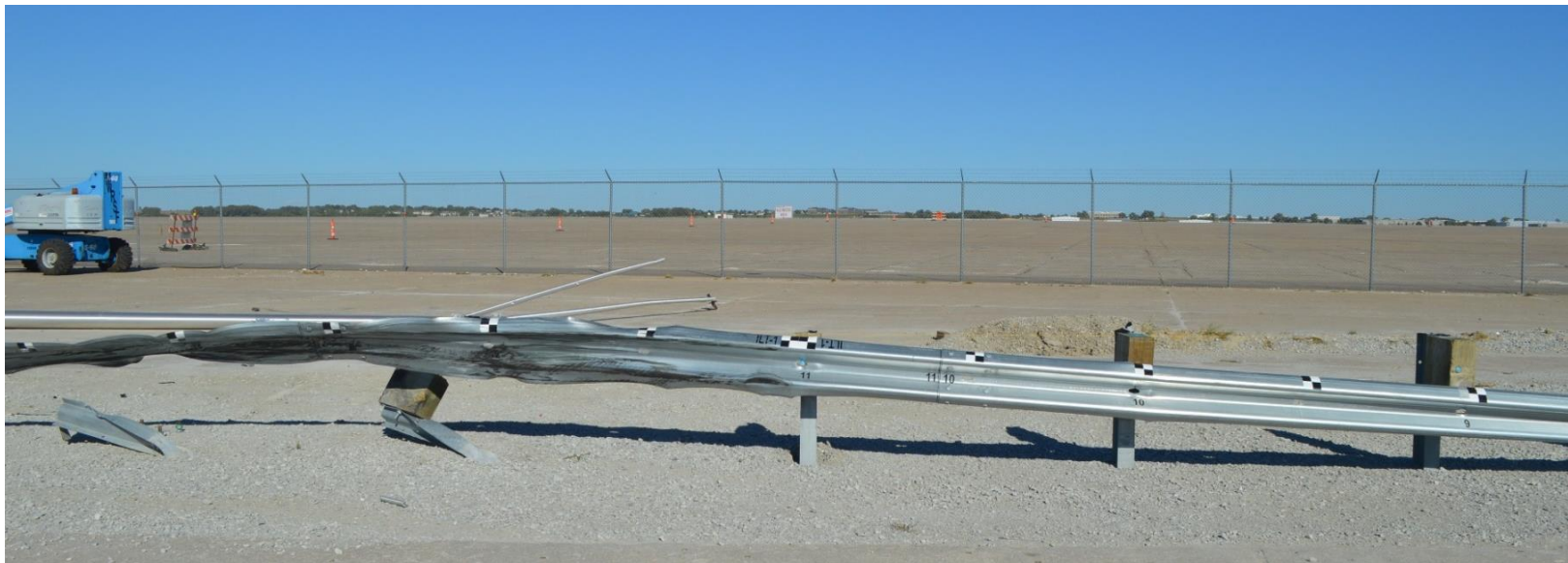
Figure 115. System Damage, Post Nos. 8 through 14, Test No. ILT-1
