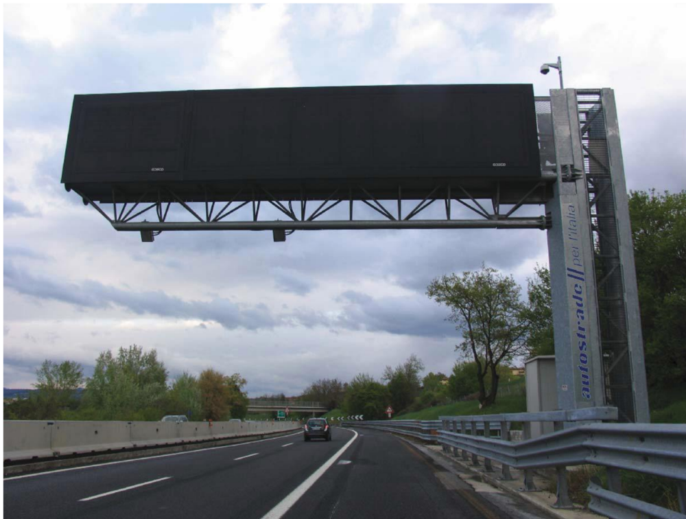
Figure 6. Sign Support and Guardrail
