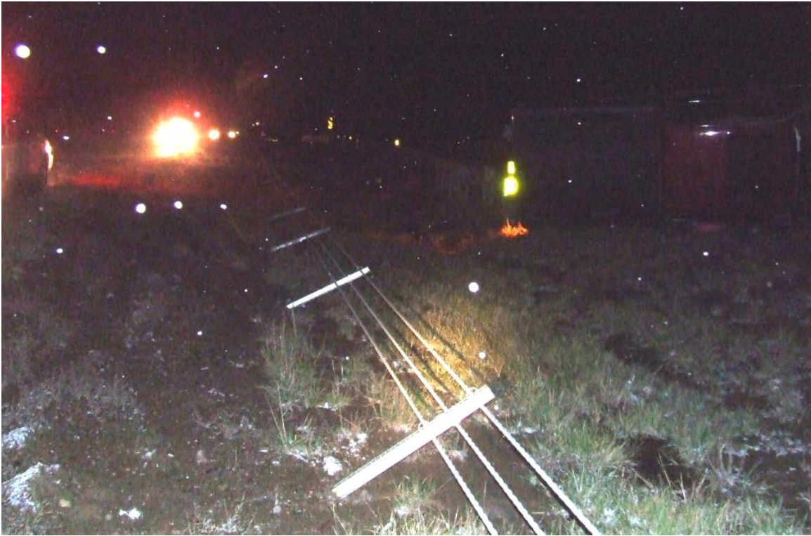
Figure 86. Penetration Crash Caused by Strong Cable-to-Post Attachment
