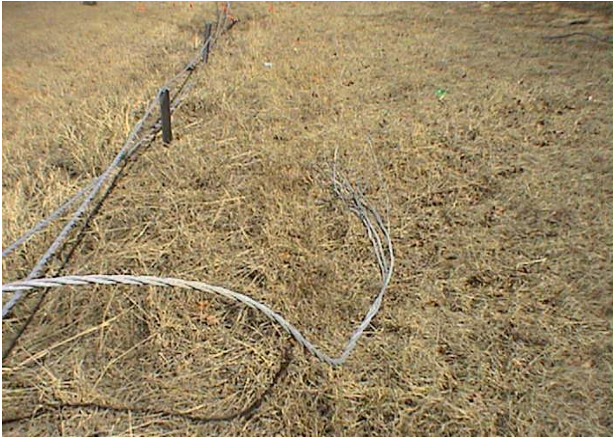
Figure 107. Splice Failure Penetration
