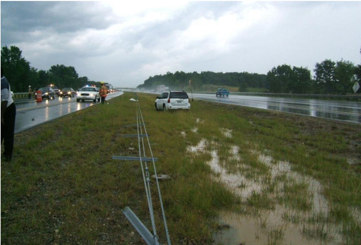
Figure 88. Override Penetration Crash Caused by Strong Cable-to-Post Attachment
