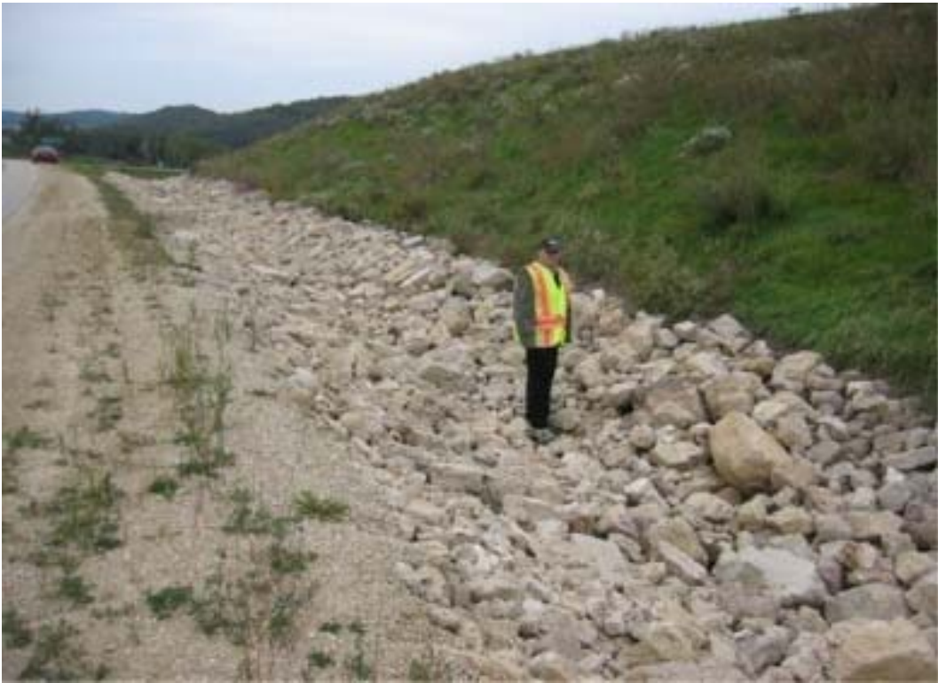
Figure 1. Roadside Rock Check Dams (above) and a Rock Ditch Liner (below)
