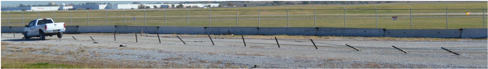
Figure 49. System Damage, Test No. MWP-4
