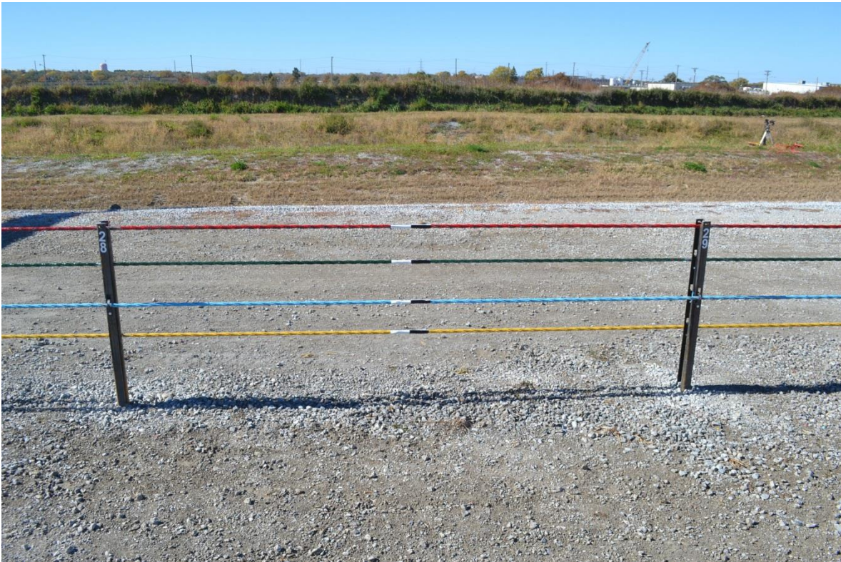
Figure 38. Test Installation Photographs, Test No. MWP-4
