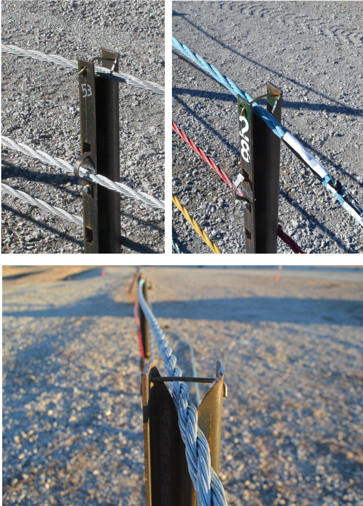
Figure 99. Example System Damage, Brass Rods, Test No. MWP-6
