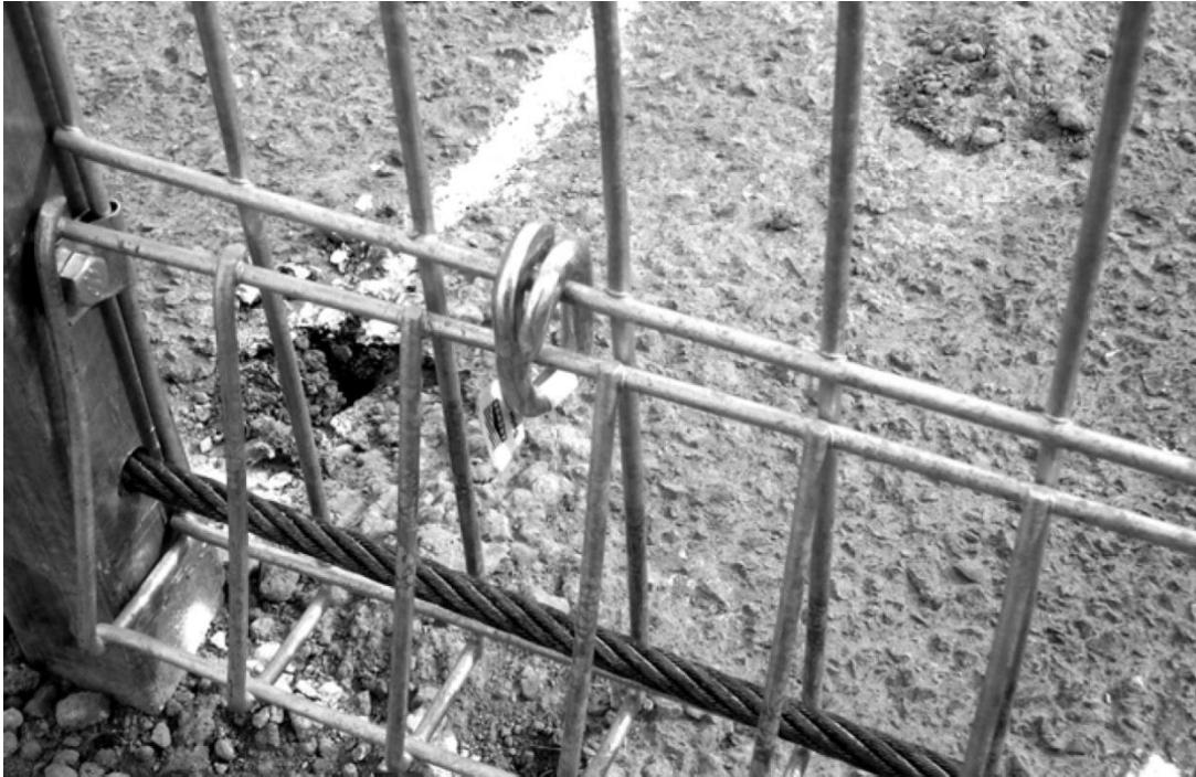
Figure 12. RTA Modified Steel Mesh [25]
