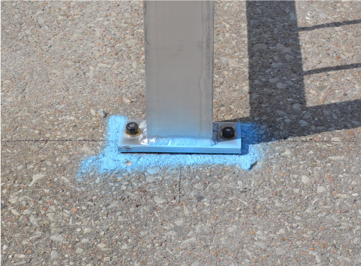
Figure 128. System Panels and Anchor, Run No. WIPR-1
