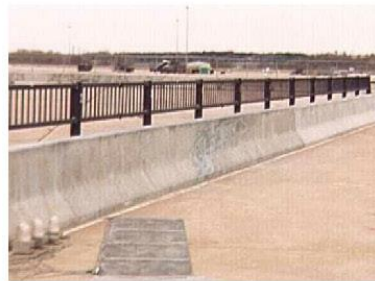
Figure 4. Concrete Traffic/Pedestrian Rail
