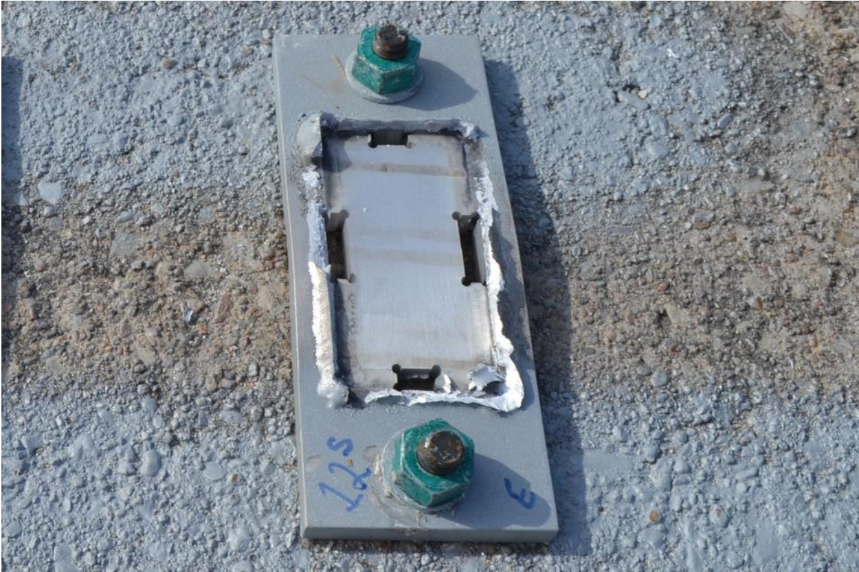
Figure 174 Slots Cut in Baseplates to Aid in Rail Fabrication
