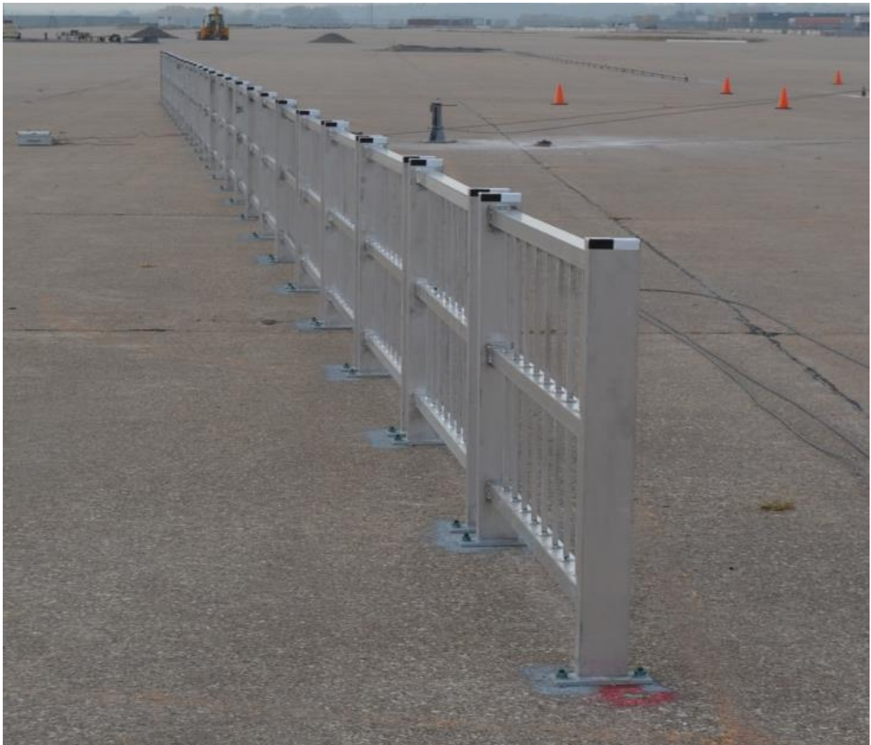
Figure 172. Pedestrian Rail Test Installation
