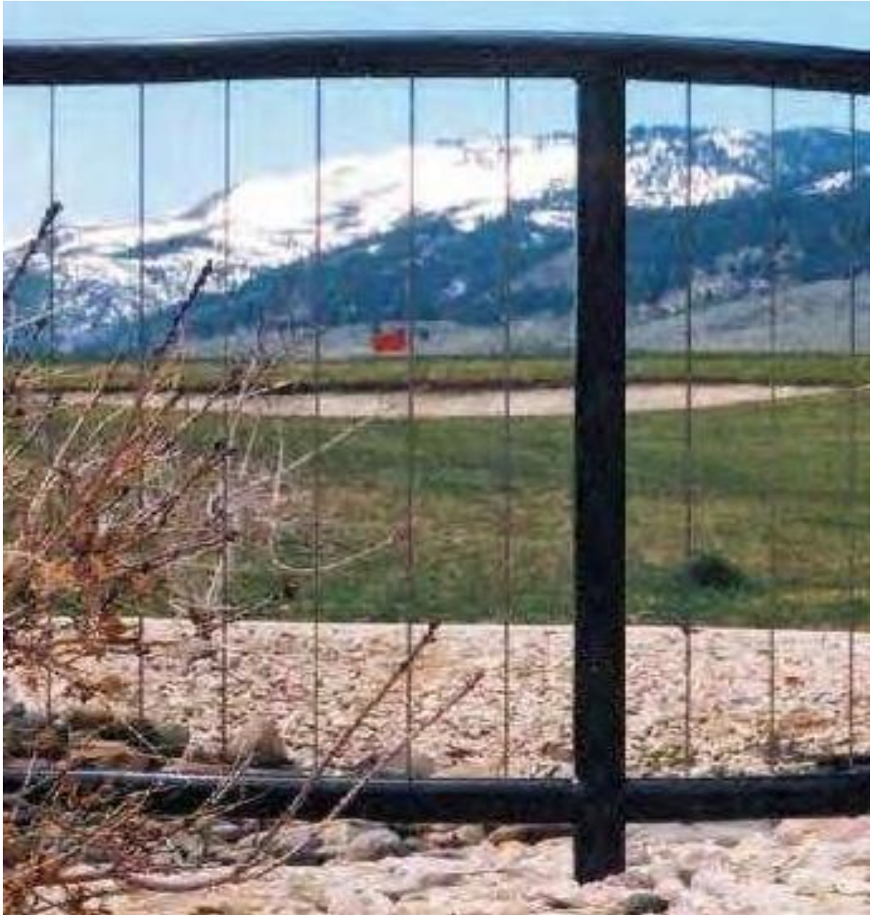
Figure 19. Vertical Cable Frame [31]
