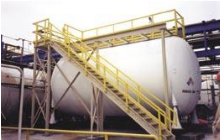
Figure 8. Examples of Existing FRP Handrail Systems [15-17]
