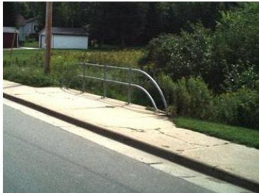
Figure 1. Rail over Culvert
