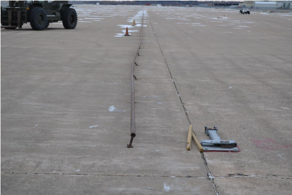
Figure 127. System Damage, Test No. IRA-4
