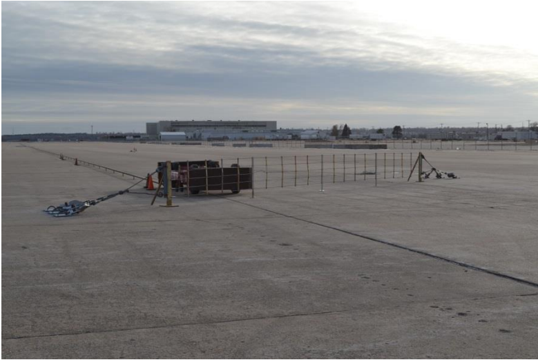
Figure 116. Impact Location, Test No. IRA-3
