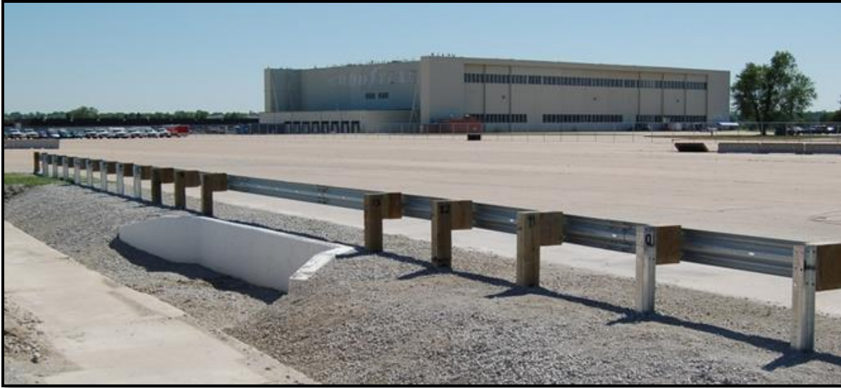
Figure 1. Midwest Guardrail System 25-ft Long-Span Design
