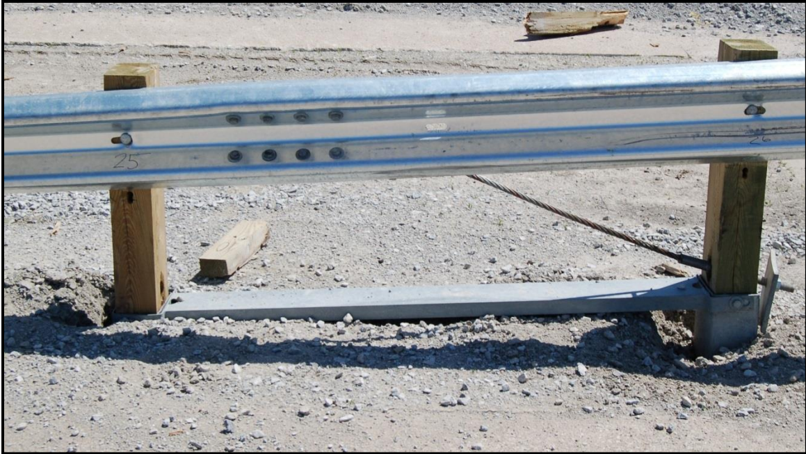
(a) Downstream Anchor, Test No. LSC-1
