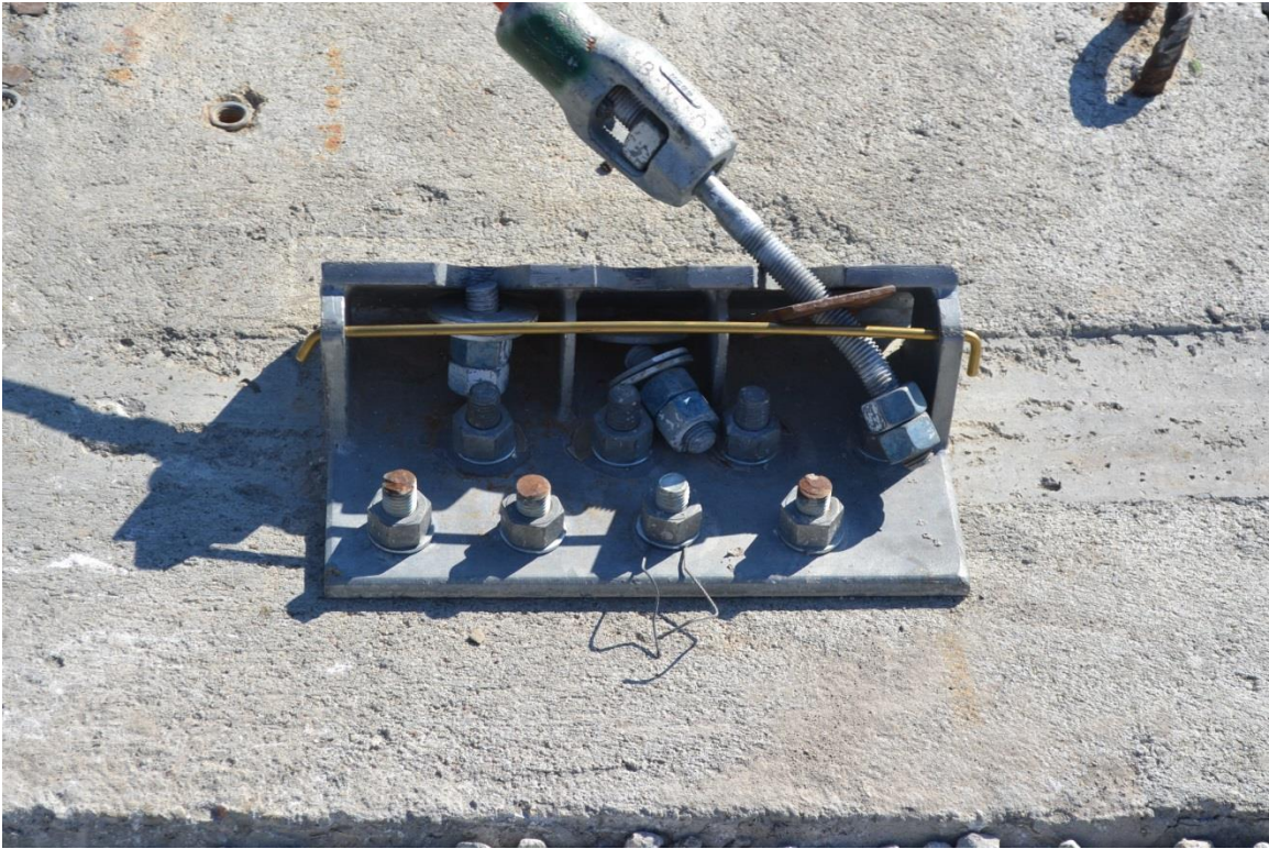
Figure 95. Downstream Anchor Damage, Test No. NYJ-3
