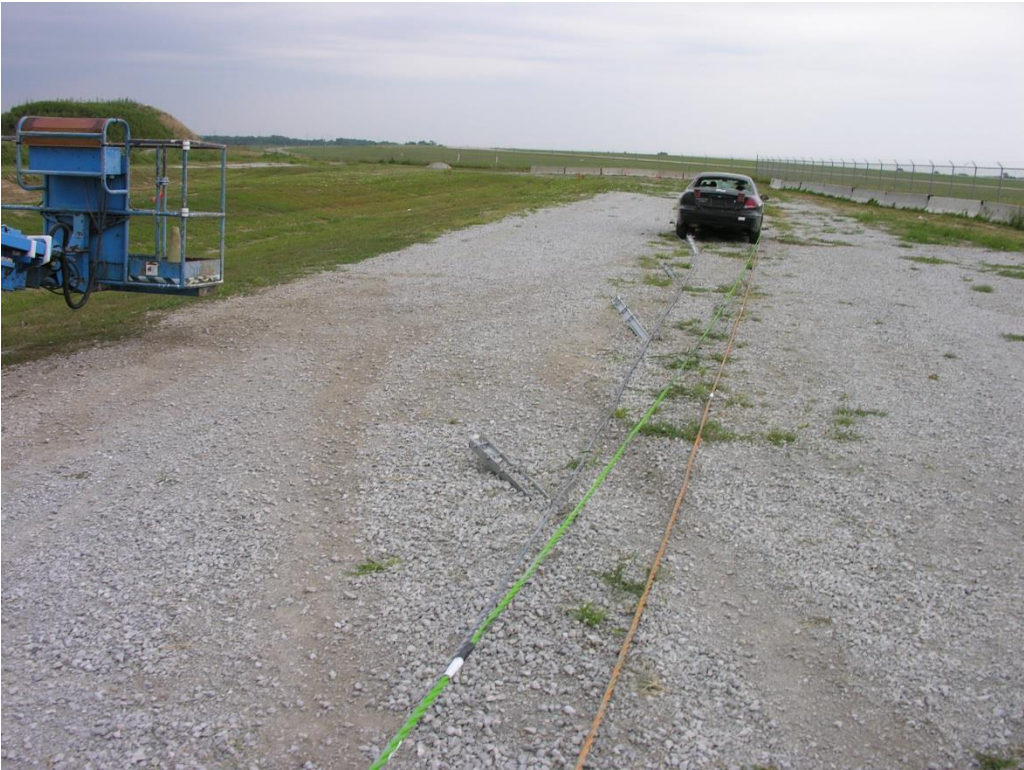
Figure 81. Post Damage in Impact Region, Test No. NYJ-2
