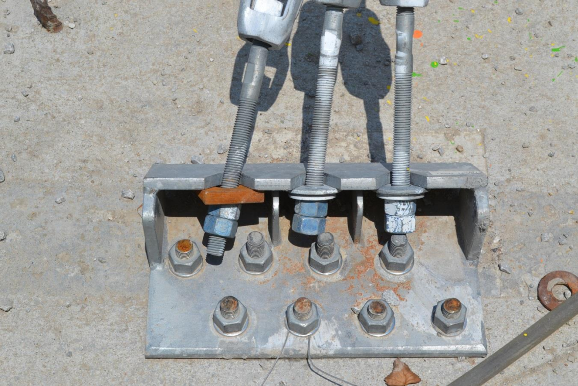
Figure 39. Upstream Cable Terminal Photographs, Test No. NYJ-1
