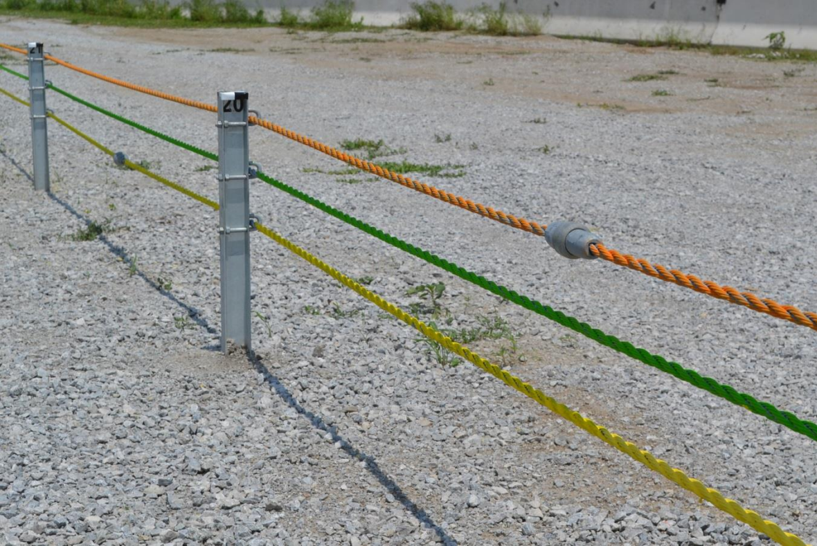
Figure 37. Additional System Photographs, Test No. NYJ-1
