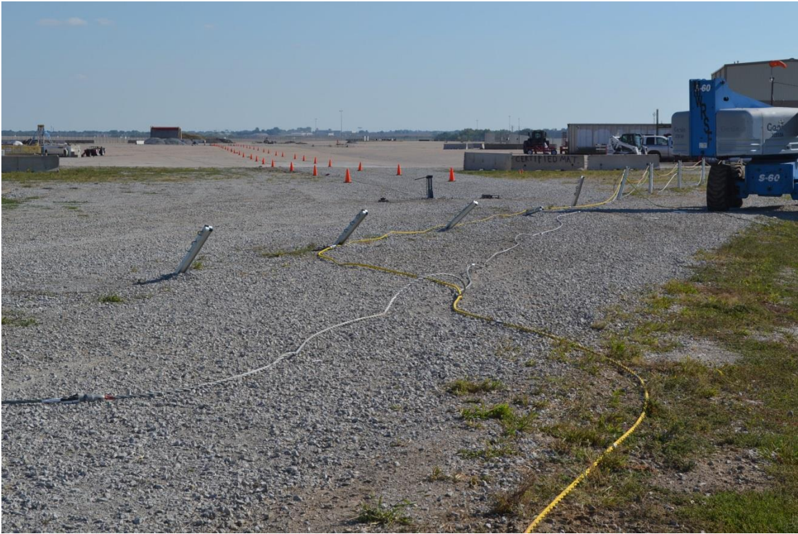
Figure 96. Post Damage in Impact Region, Test No. NYJ-3
