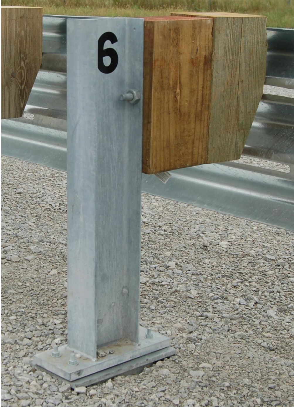
Figure 1. UBSP Installed in the Thrie Beam Bullnose
