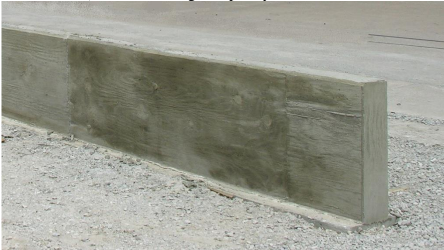
b) Permanent Concrete Barrier
