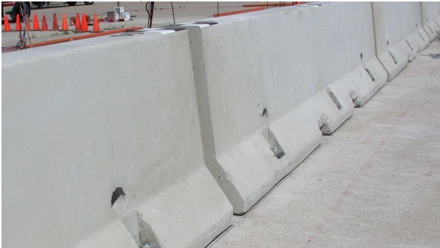
c) Temporary Concrete Barriers with Restrained Movement
