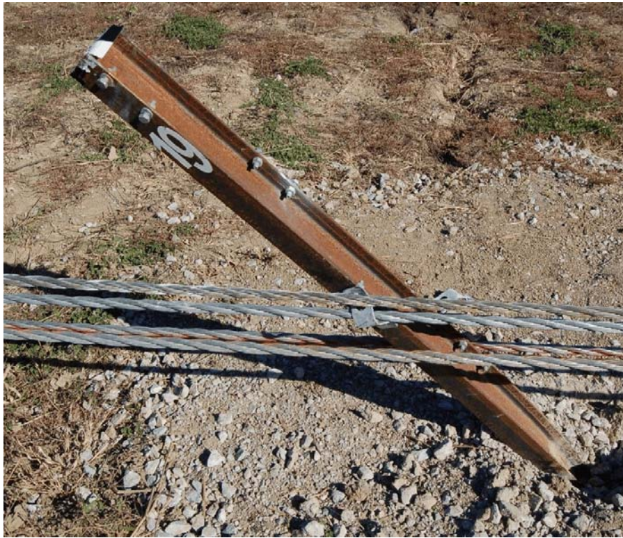
Figure 42. Posts Nos. 17-19 Damage, Test No. 4CMB-1
