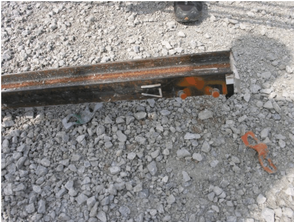
Figure 107. Post No. 17 Damage, Test No. 4CMB-3
