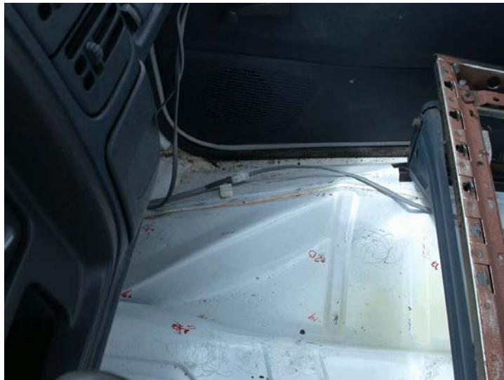
Figure 59. Occupant Compartment Deformations, Test HTB-2
