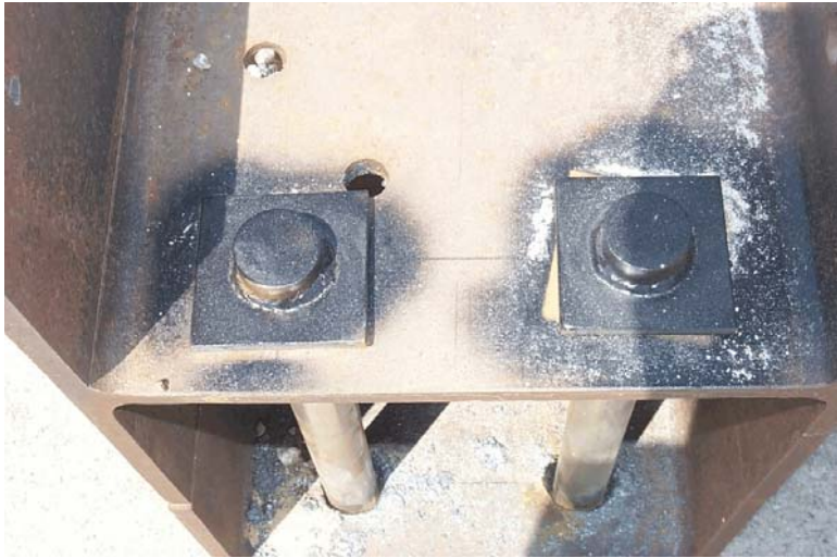
Figure 6. Splice Details for Steel H-section Temporary Barrier
