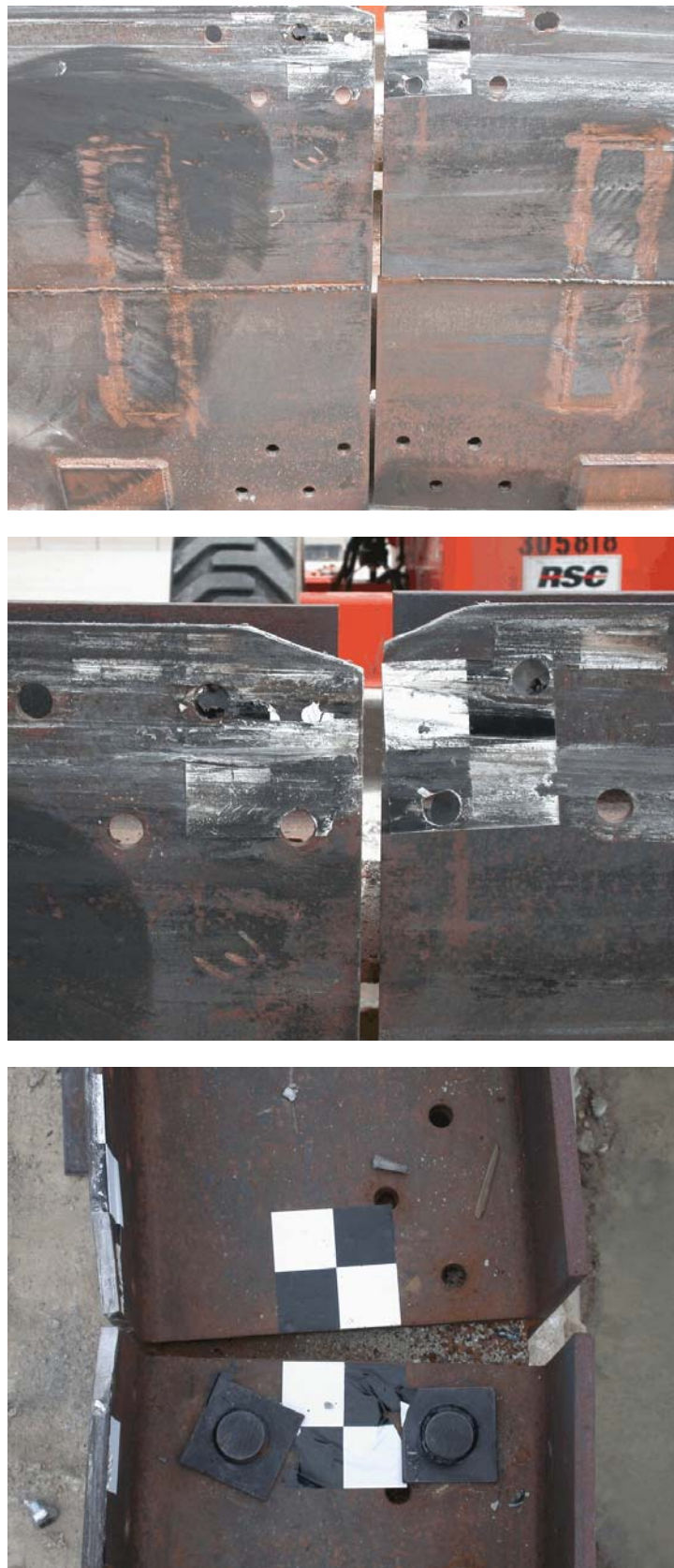
Figure 52. Splice Rotation and Damage, Test HTB-2
