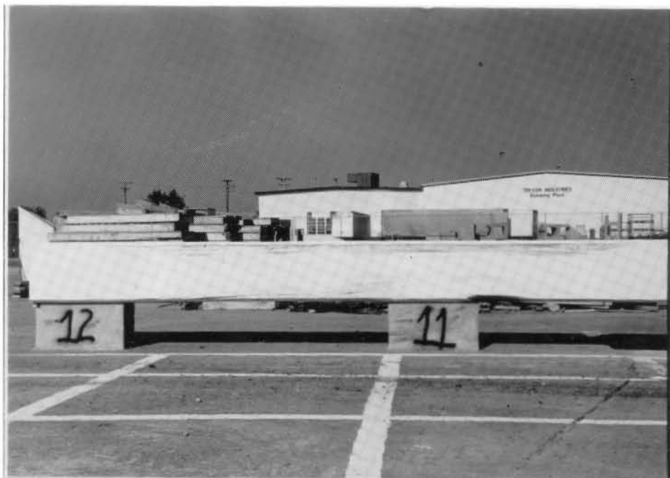
FIGURE 34. Bridge Rail Damage of Second Impact, NEOCR-1
