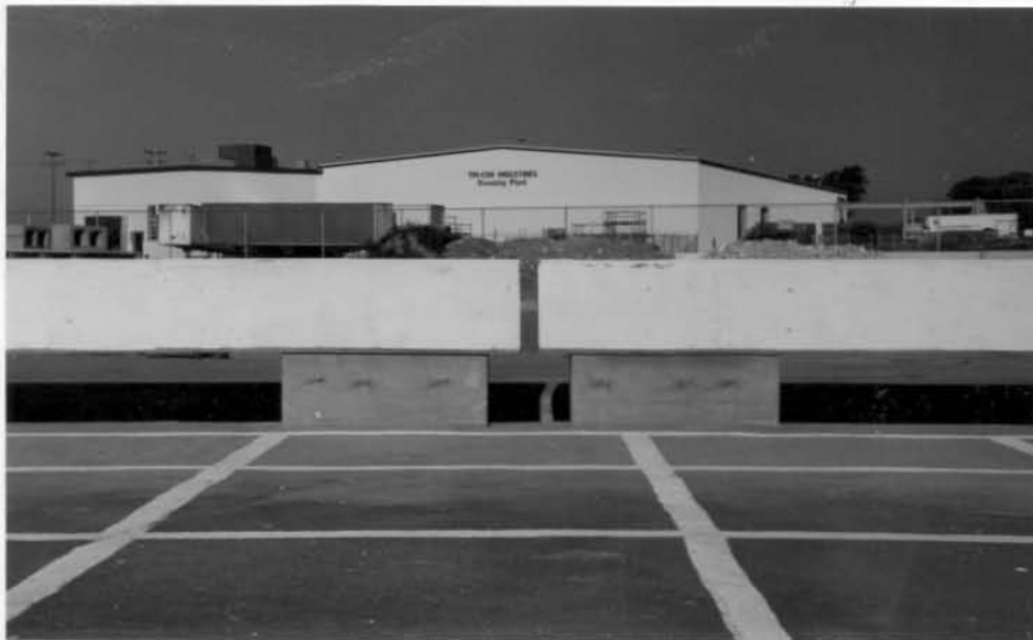
FIGURE 16. Nebraska Open Concrete Bridge Rail
