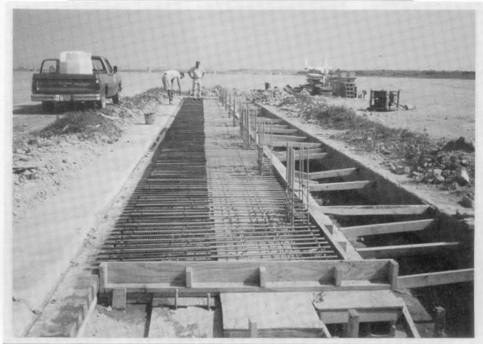
FIGURE 18. Reinforcement Layout for Bridge Deck
