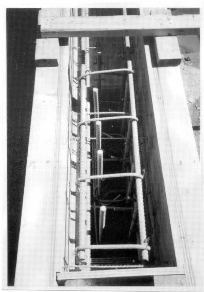
FIGURE 19. Steel Reinforcement in the 3-ft Posts Adjacent to the 3-in. Gap
