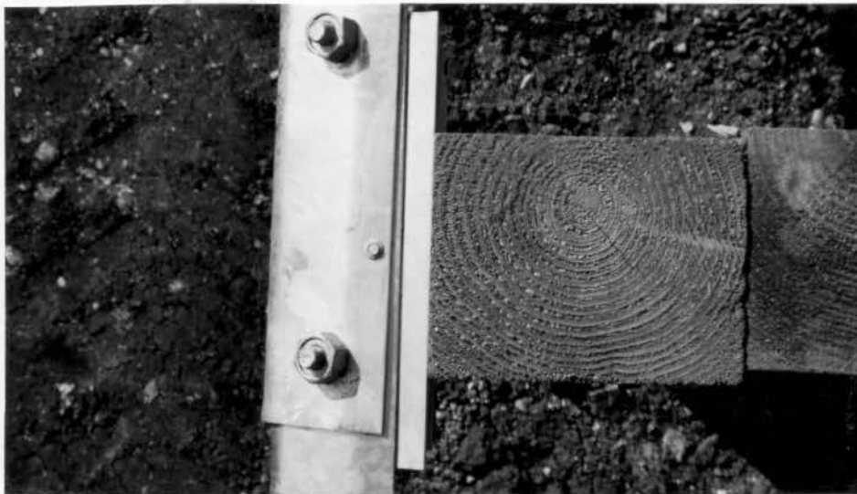
FIGURE 6. Guardrail Connection Detail, Post No. 3
